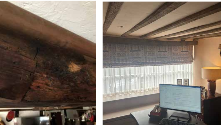
Photographs of oiled oak joist prior to restoration Photographs of ground floor study - previously not visible timber frame on ceiling exposed
