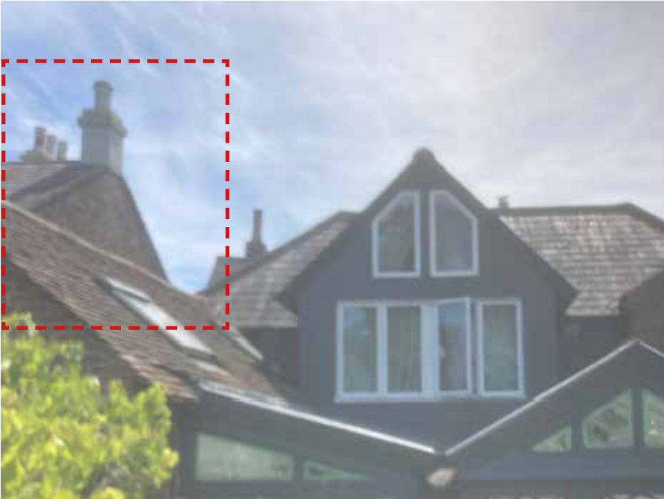
109 High Street south gable wall before re-pointing
