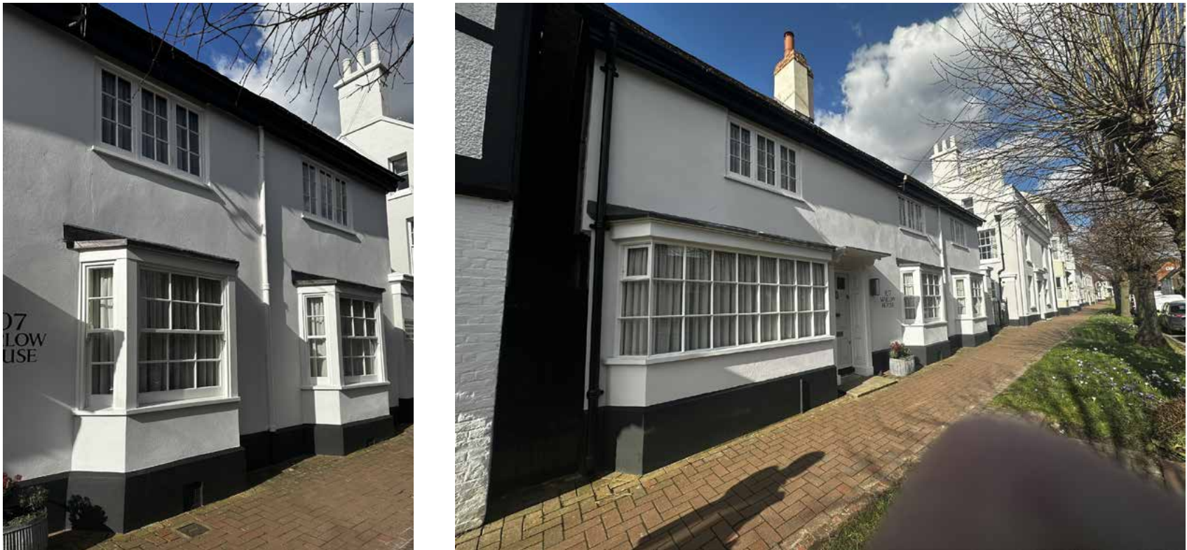
Photographs of front elevation after restoration works
