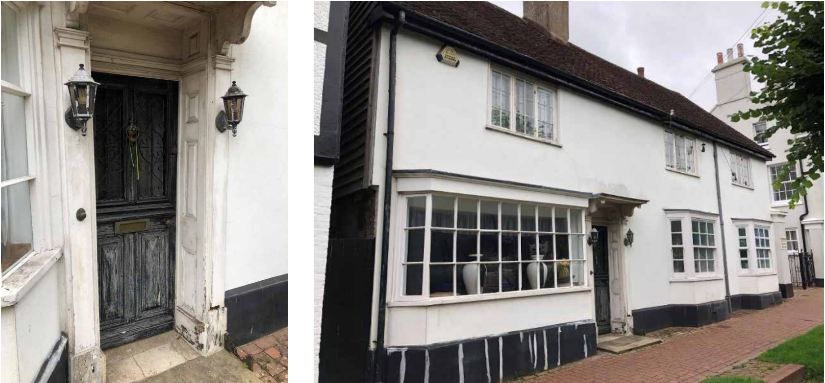
Photographs of front elevation before restoration works
