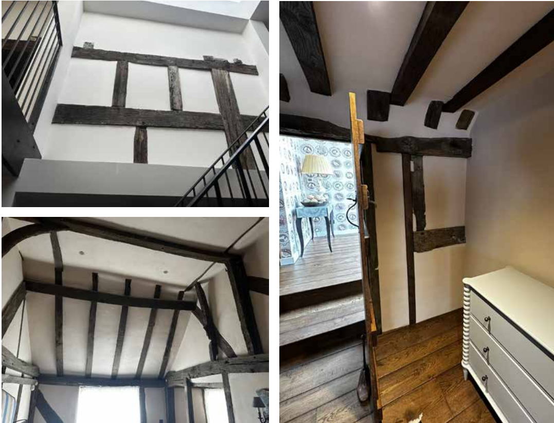
Photographs of restored historic oak frame
