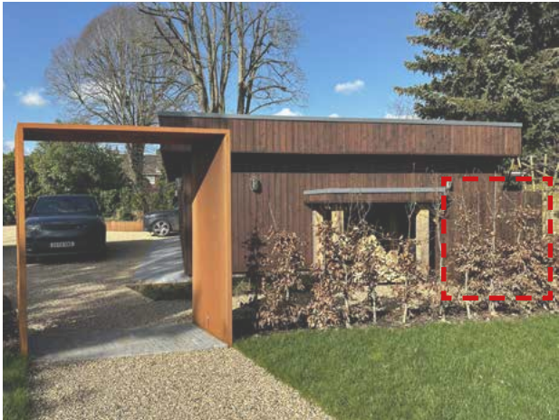
Recent photographs of the irrigation tank enclosure
