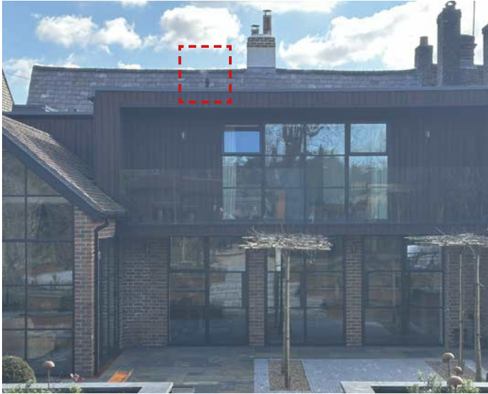
Recent photograph capturing the new boiler flue
