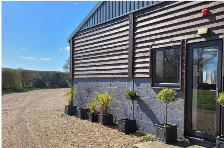
The materials to be used in the new barn will match those of the existing barn. The walls will be horizontal stained feather edge boarding over painted concrete block walls. The doors and windows will be grey upvc and the roof will be profile roof sheeting in merlin grey.
