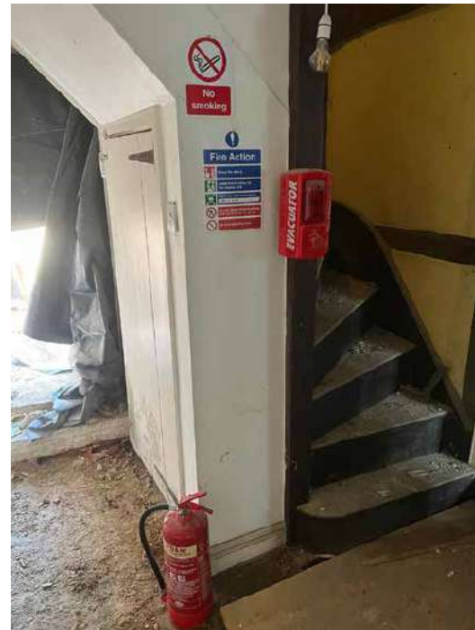
Staircase during demolition works
