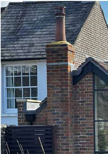
Recent photograph of parapet wall detail
