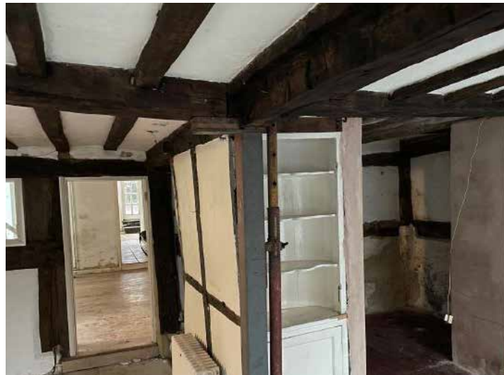
Internal wall and steel beam before removal
