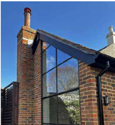
‘As-built’ bake house chimney with lead waterproofing dressing
