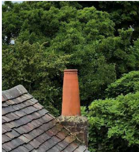
Original bake house chimney
