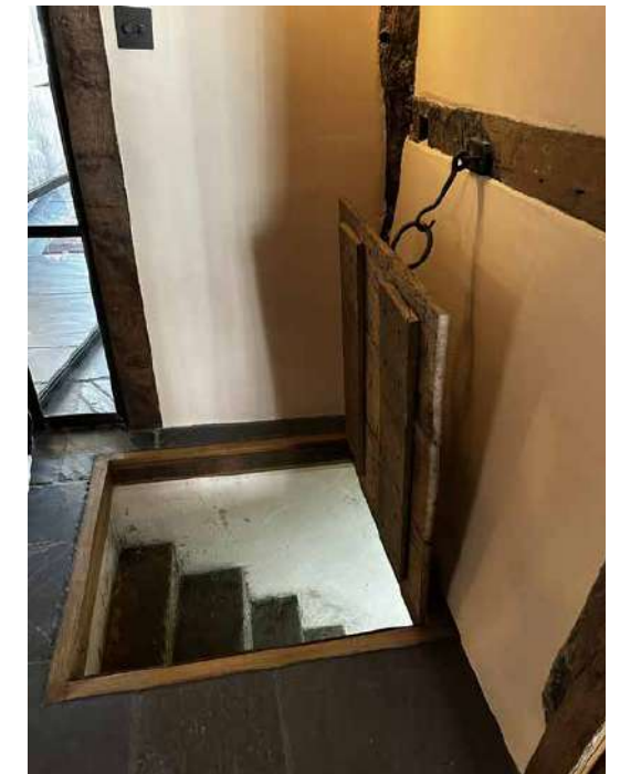
Current photograph- staircase removed, trap door to basement access made out of historic floorboards and installed
