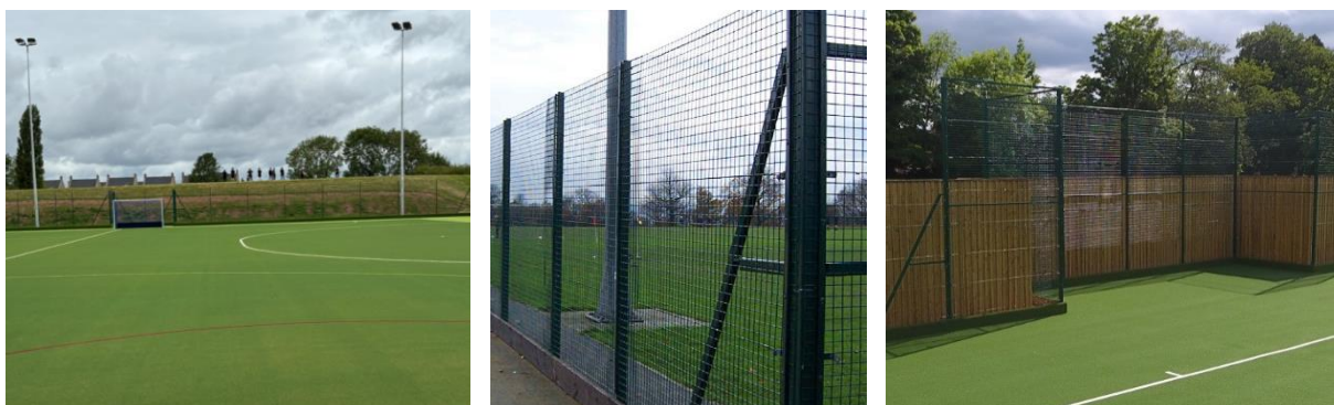
Figure 4: Images of a typical artificial turf with floodlights (left), mesh fence (centre), and acoustic barrier (right)
