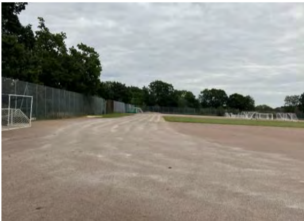
Figure 2-B: View across the existing running track; looking east along the northern boundary.
