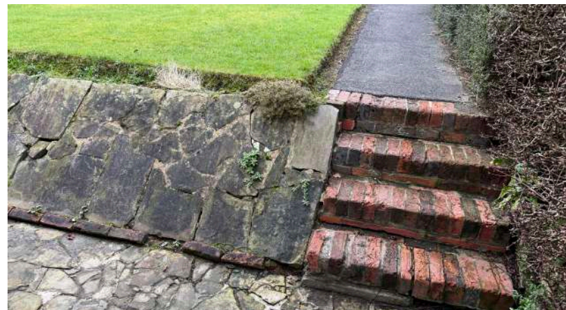
raked wall, path and steps to be replaced
