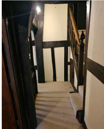
stair to first and attic floor
