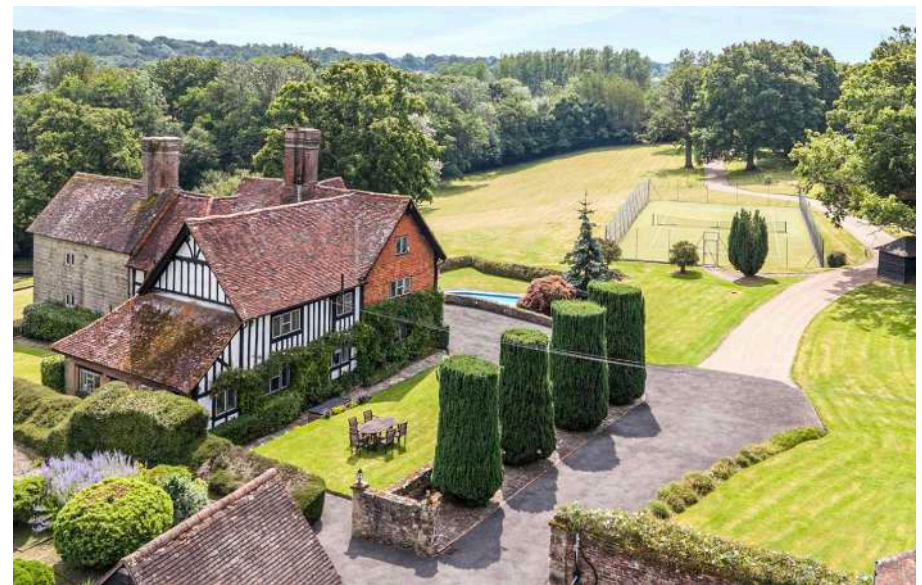
west elevation showing sports pitch and coachhouse to the northwest
