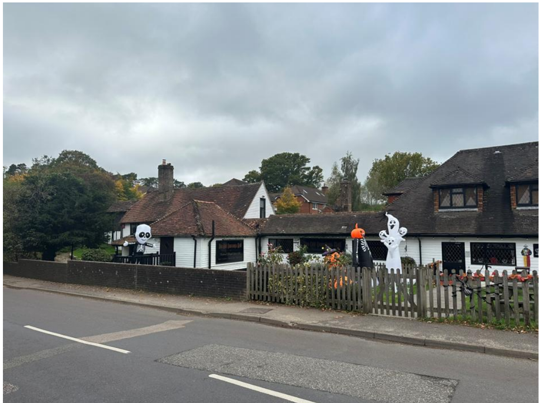
Figure 8: Dunnings Mill viewed from West Hoathly Road. The original building is visible to the left, with the various one and two storey extensions to the right (north). Recent development at Streatfield Place, which is elevated above the Mill, is visible in the background.
