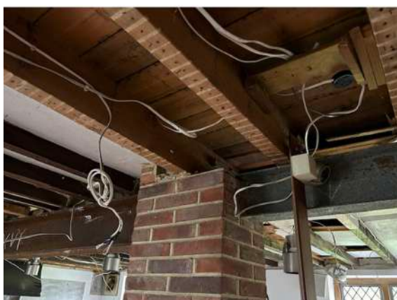
C20th timbers and inserted steel beams and brick pier
