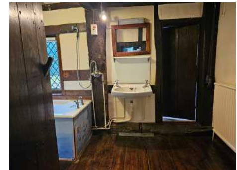
Bathroom to bedroom 1
