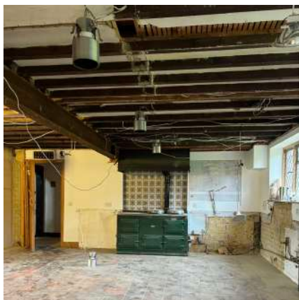
modern timber boarding to ceiling removed to expose original ceiling
