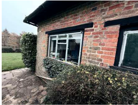
view of north elevation and windows to be replaced
