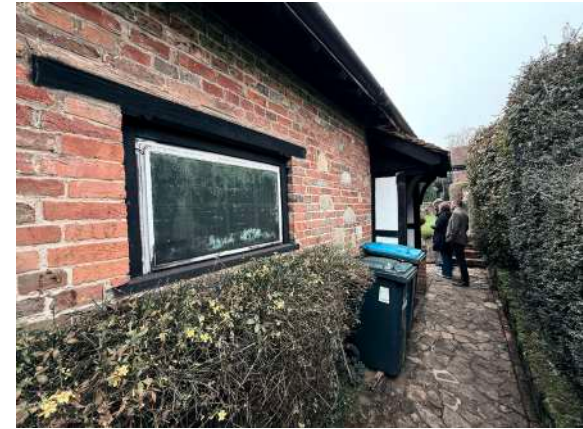
view of north elevation and windows to be replaced and porch to be repositioned and paving to be replaced
