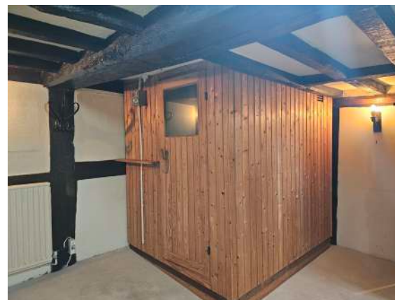
sauna to be removed to 1st floor bathroom
