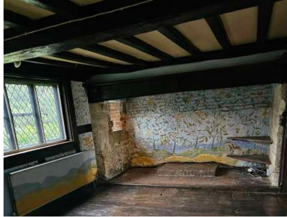
fireplace in rear reception room to receive wine fridge
