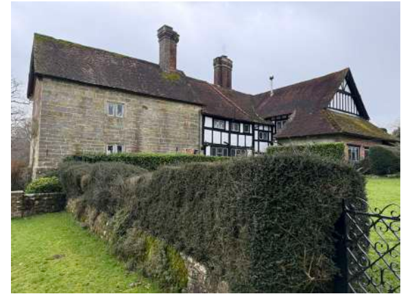
view of north elevation showing lean-to roof to receive rooflights
