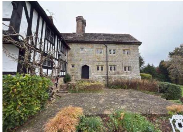
view of south terrace and paving to be replaced
