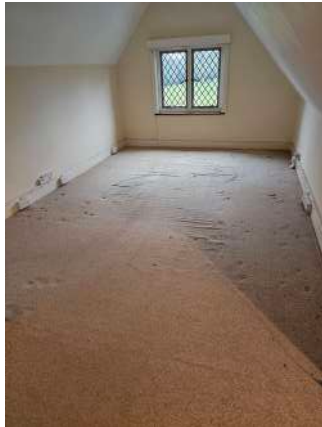
south gable attic bedroom to 2nd floor of C17th range
