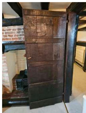
original C17th ledge and boarded door to be matched in C20th range
