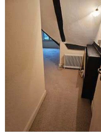
modern partition to 2nd floor to be repositioned
