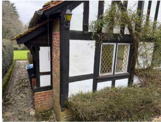
window to be replaced
