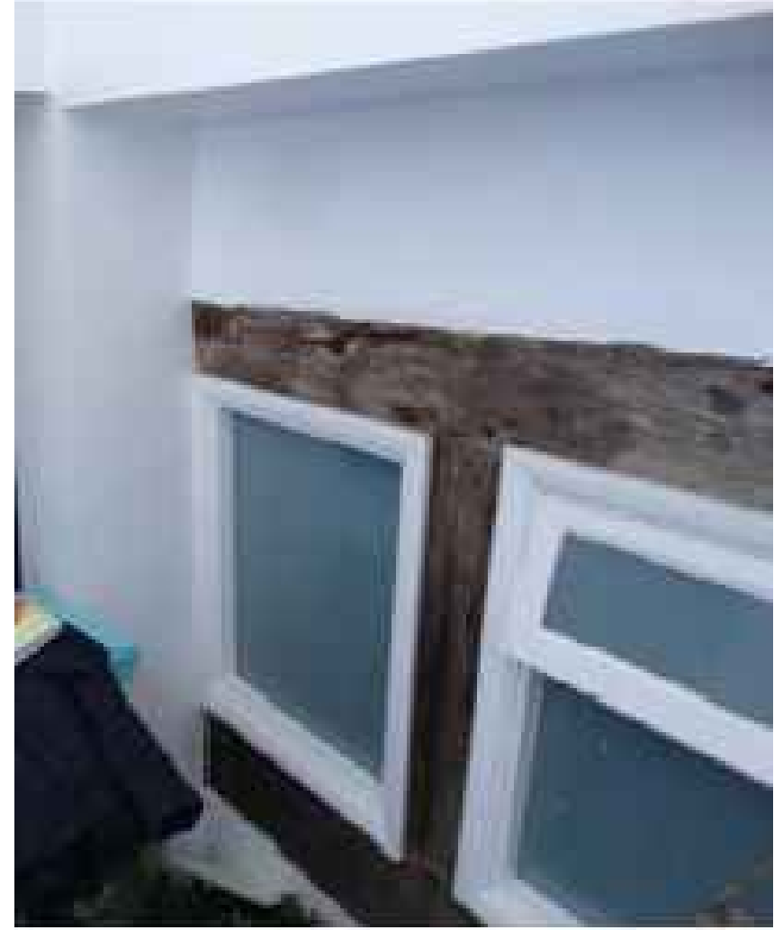
Before: uPVC casement windows before removal
