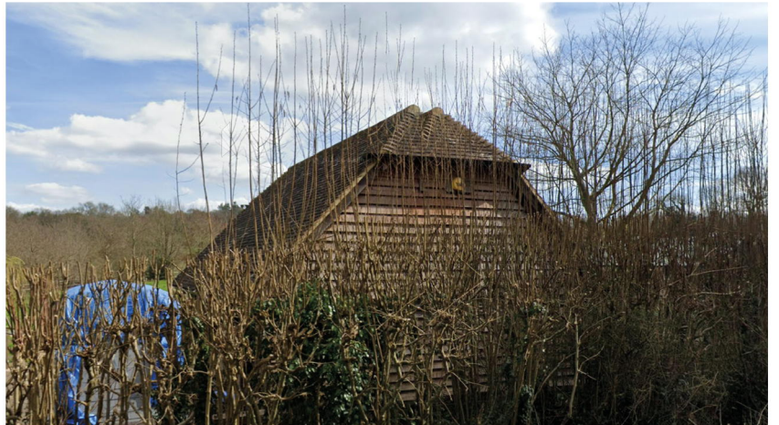
Fig. 6. Another example of horizontally installed, timber cladding on Brook Street (Google Maps).
