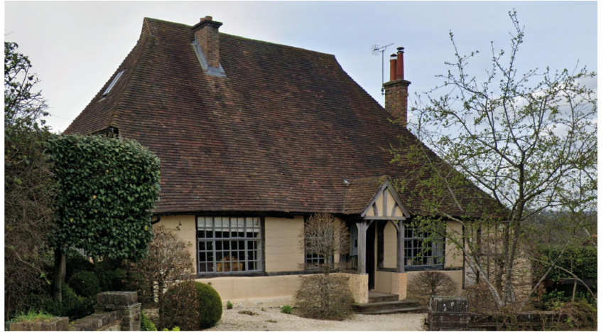
Fig. 8. Traditional render-like finish to a property facing Brook Street (Google Maps).
