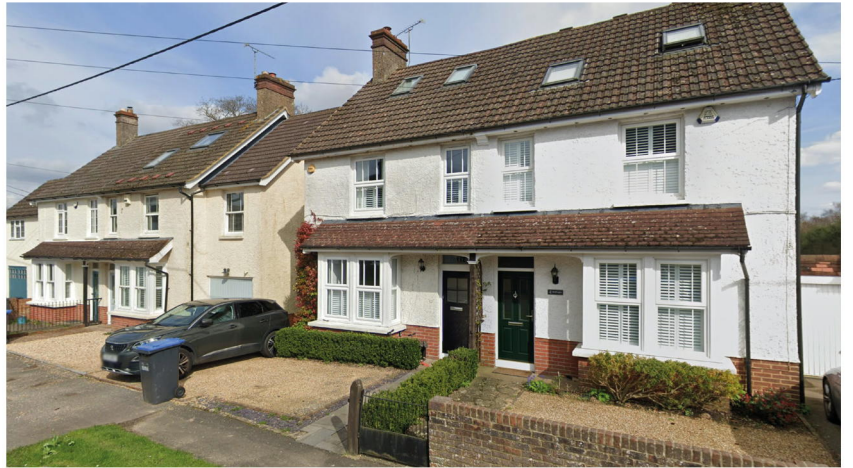
Fig. 9. View of existing properties on Brook Street with rendered façades (Google Maps).
