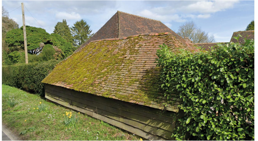
Fig. 5. Example of horizontally installed, timber cladding on Brook Street (Google Maps).
