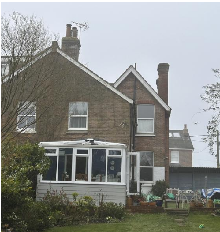
View of rear of Stonecroft with conservatory in foreground.
