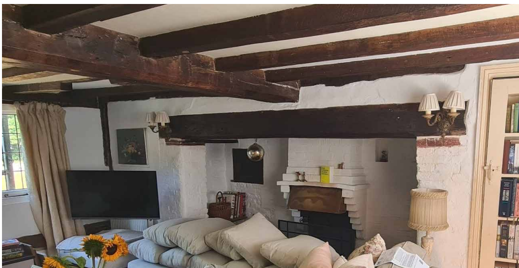
Bridging beam with false joists resting over the original inglenook's bressummer. Built-in oven left of fireplace
