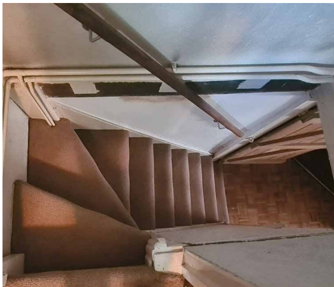
Girding beam by the stairs with signs of three cut joists and opposite reused trimmer joist with two mortices
