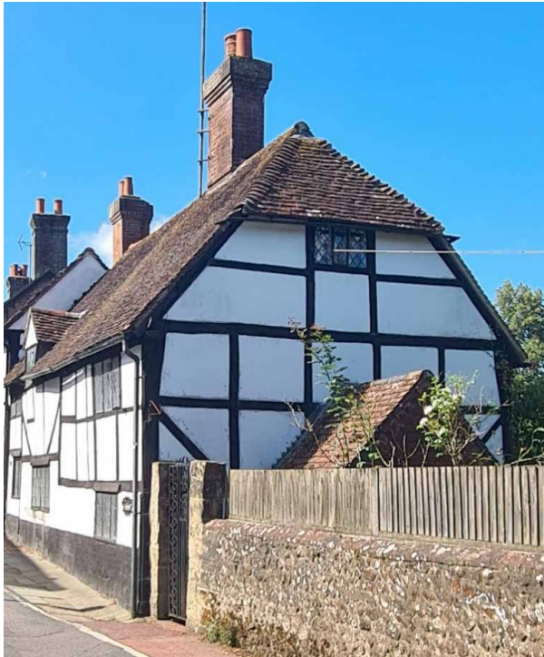
Late C18 north extension with uniform square panel cross frame gable and the Great Bricks used to make a step
