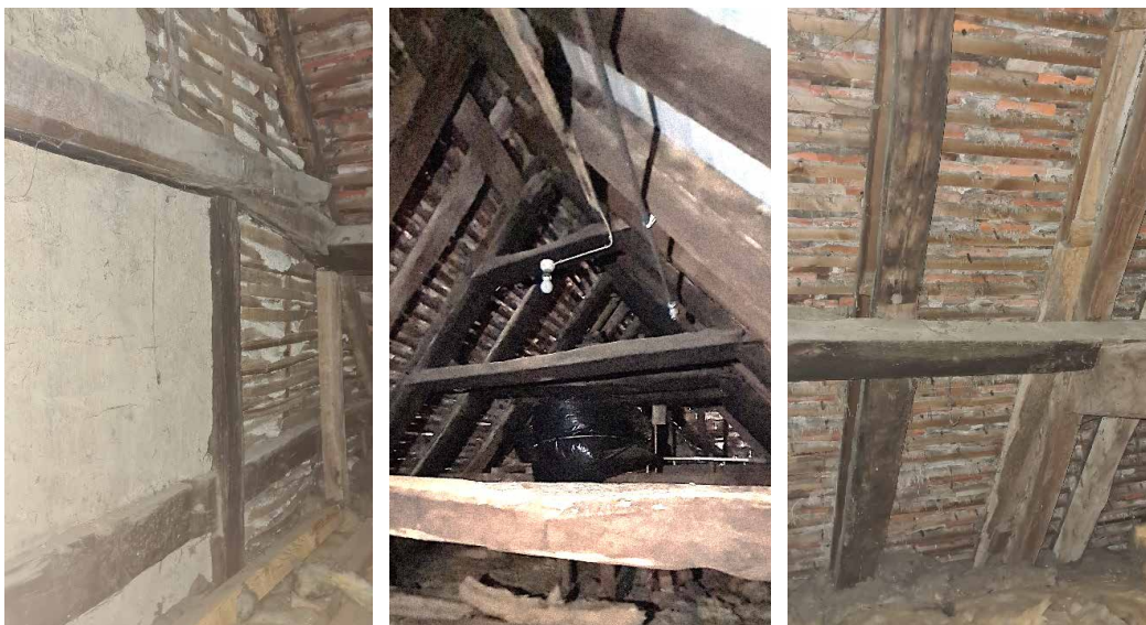
Original external wall with terminal chimney behind; Unusual middle double collar truss; Later roof structure
