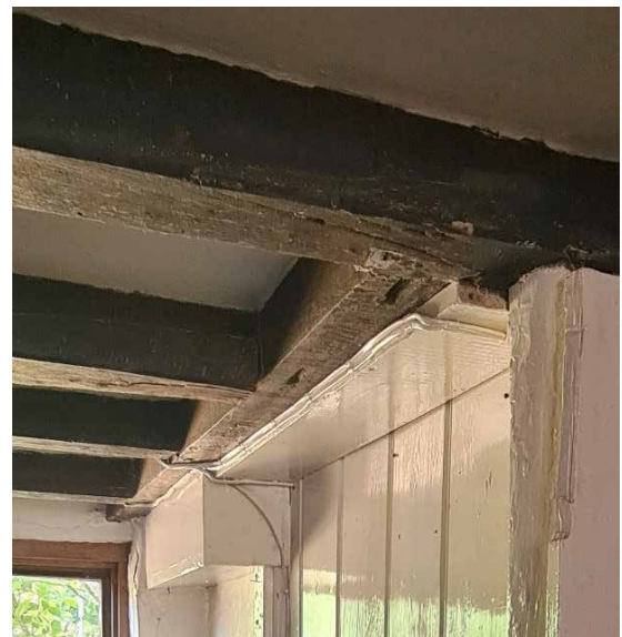
Girding beam by the stairs with signs of three cut joists and opposite reused trimmer joist with two mortices
