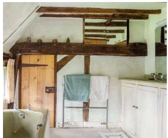
Front bay box frame construction and original angled braces on north wall frame in two rooms, one cut by the door
