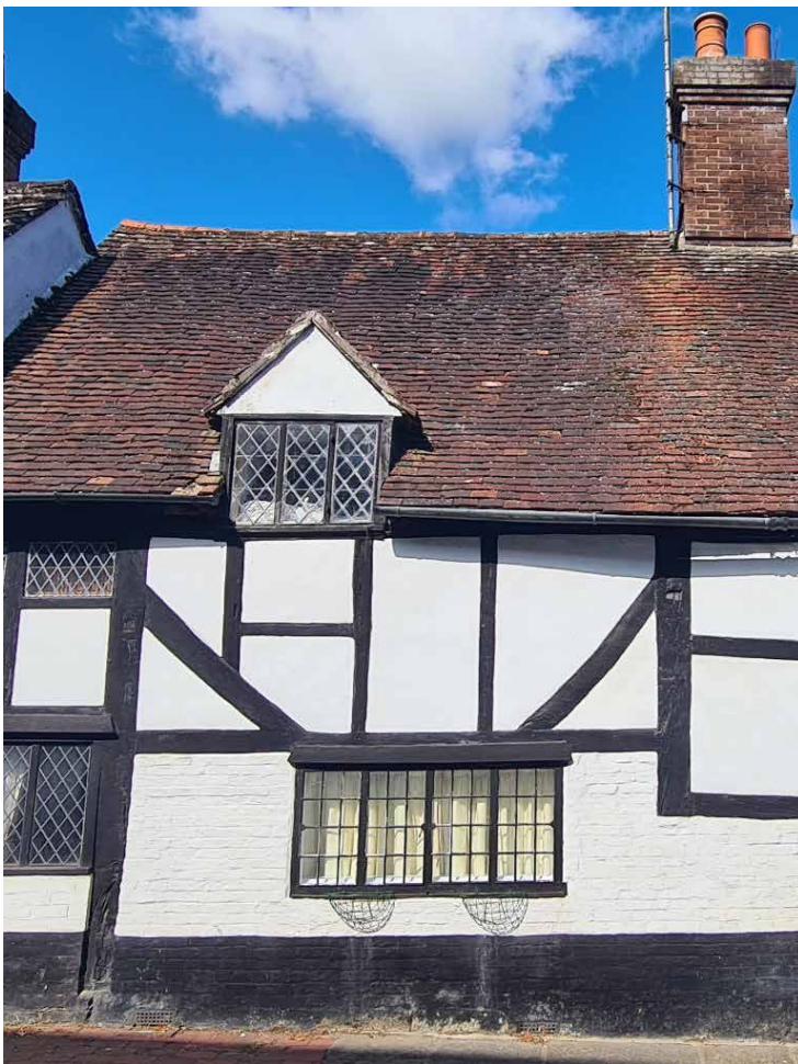
Front bay box frame construction and original angled braces on north wall frame in two rooms, one cut by the door
