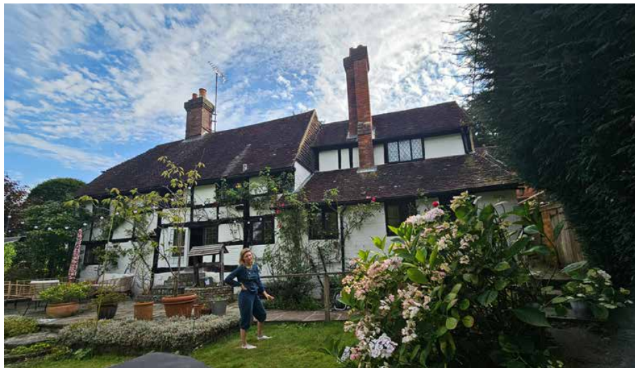
Rear view of existing house
