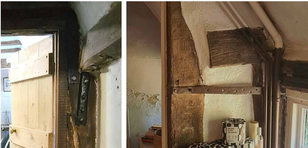
Wrought iron bracket and strap securing the new wall plate and restraining the old wall frame respectively
