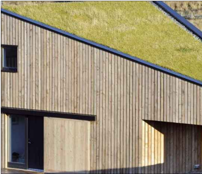
TIMBER CLADDING; PRODUCT; LARCH BOARD ON BOARD CLADDING COLOUR; 'UNCOATED', SIZE: 150mm BOARDS
