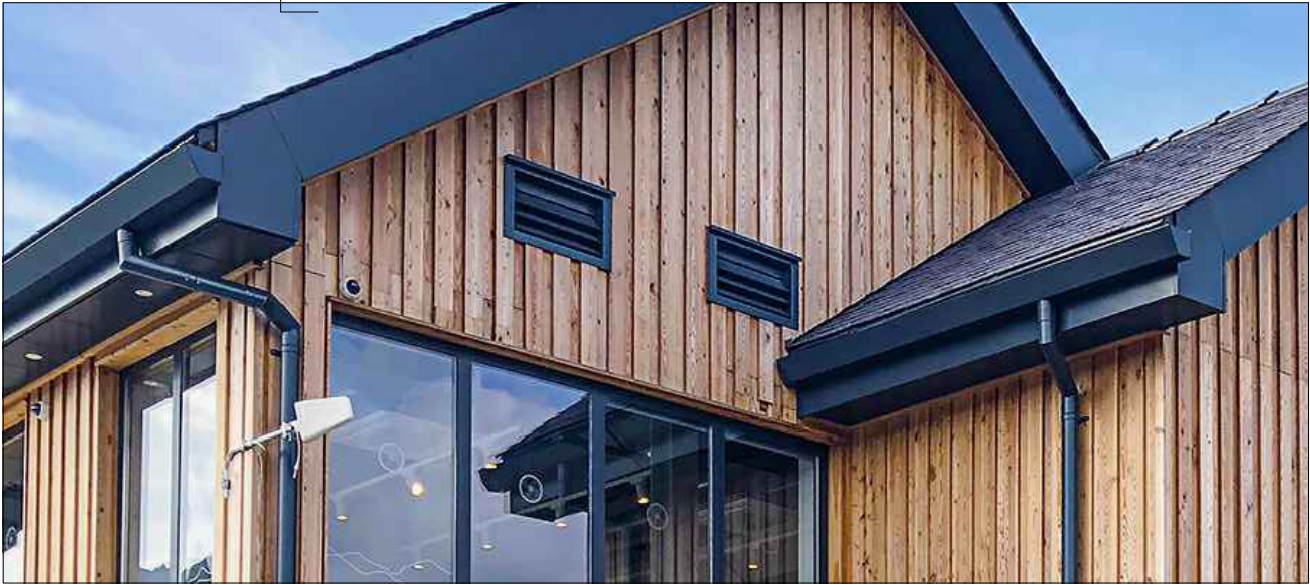
Aluminium Gutter & RWP
