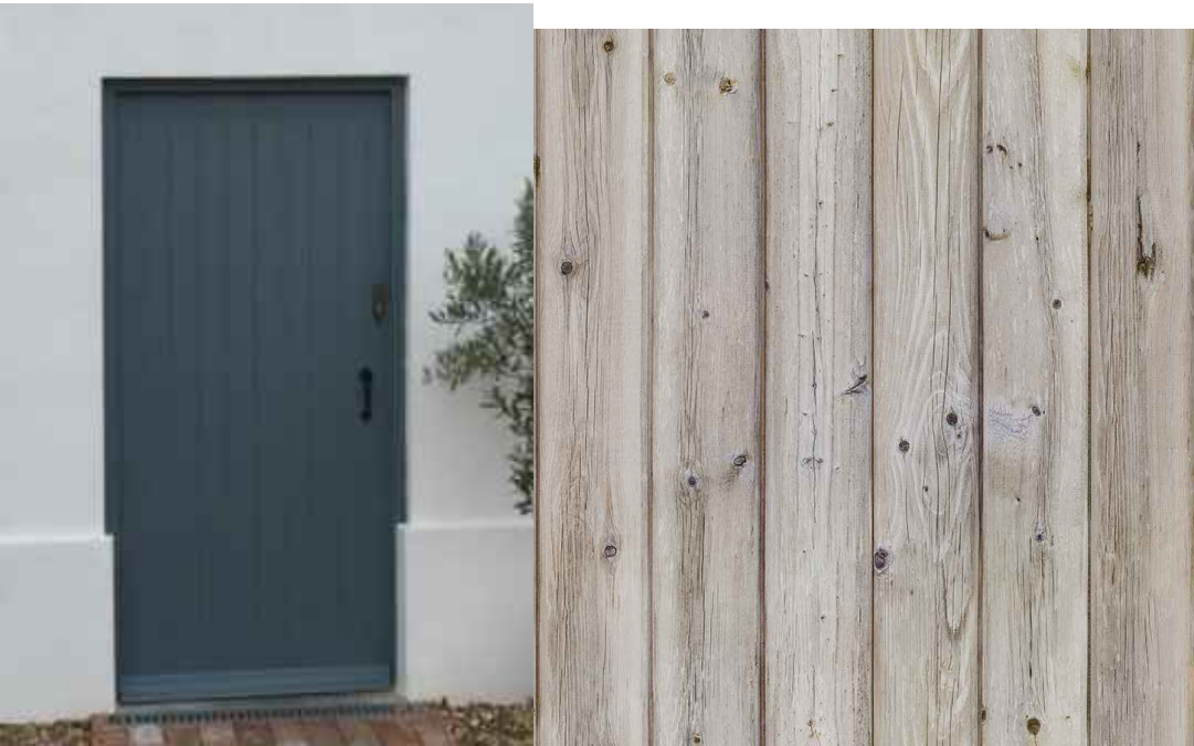
Painted timber framed doors and windows
