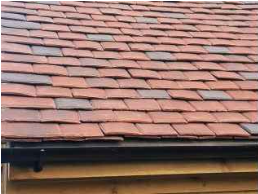
Tudor Restoration roof tiles
