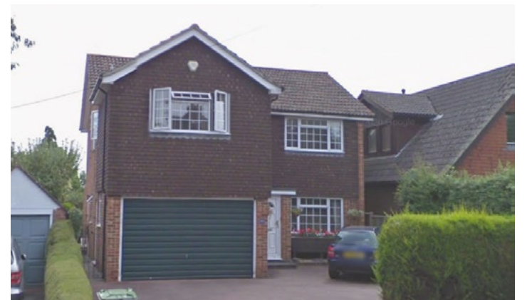
6. 123 College Ln, 2 storey, multi brick and hanging tiles
