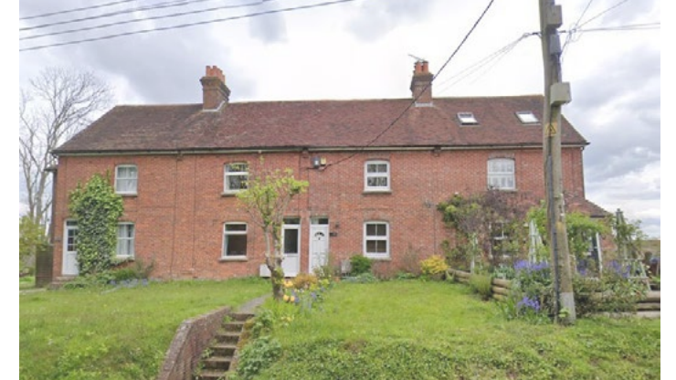
2. 163 College Ln 2 storey, red brick
