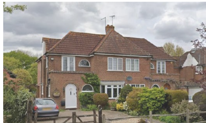
4. 114 College Ln 2 storey, red brick
