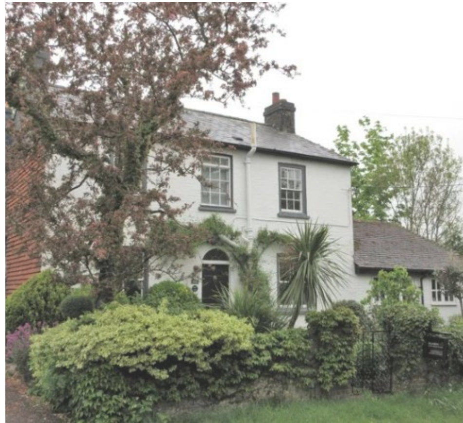
1. Listed building, Grove Cottage 2 storey, slate roof, painted brick
