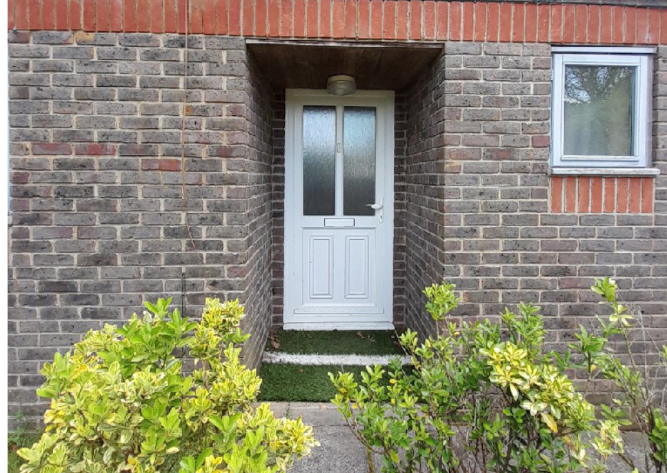
Existing Front entrance to caretakers house
