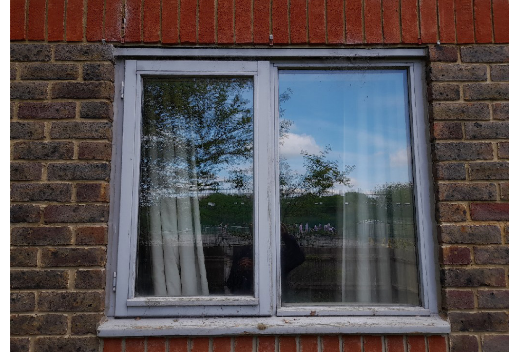
Existing windows (all windows to be replaced)
