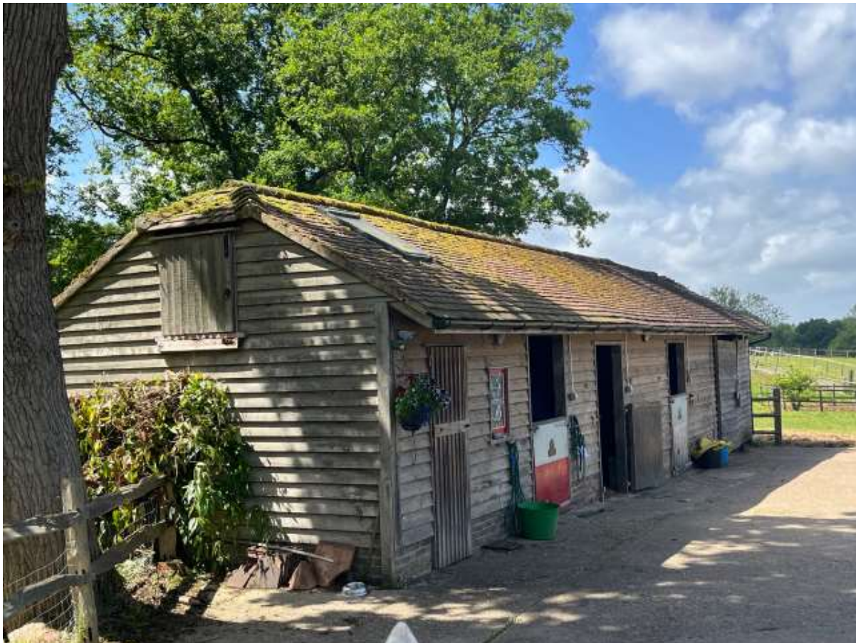
Stable building – north east elevation
