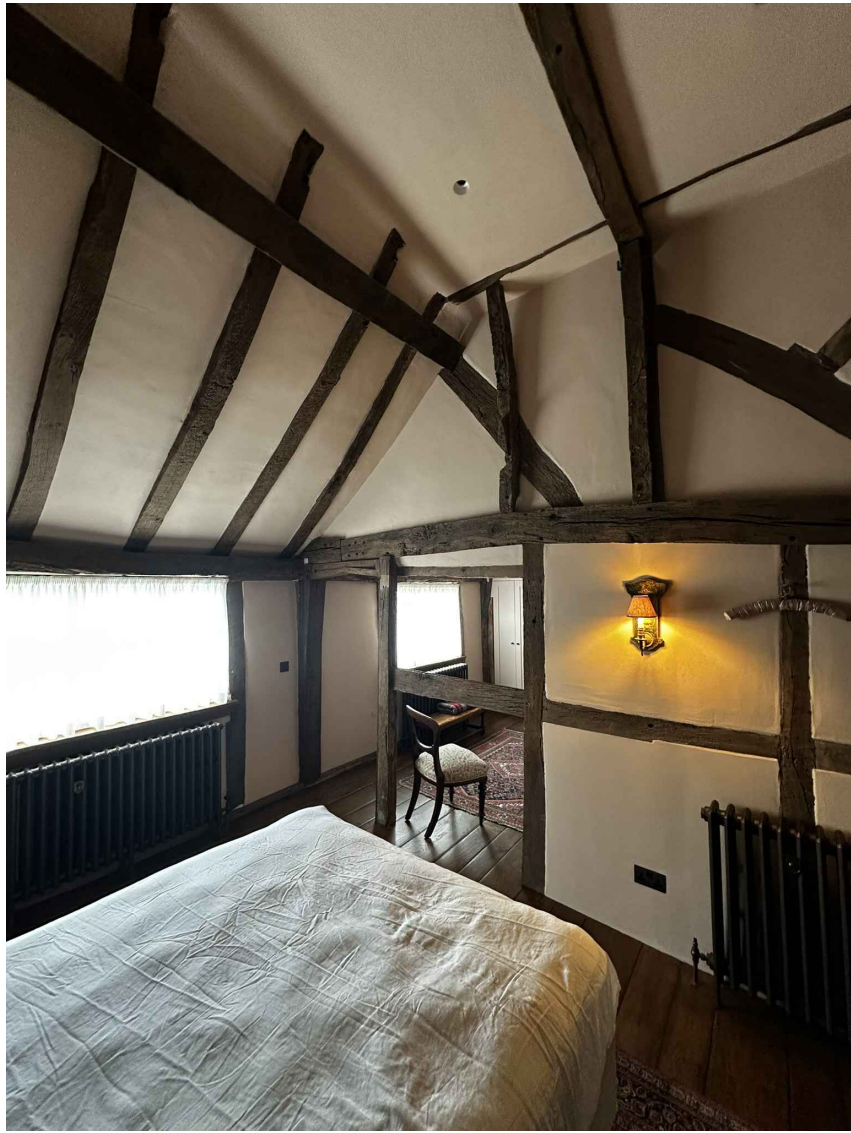
Northern bedroom - view towards wall with removed infill paneling and retained timber framing
