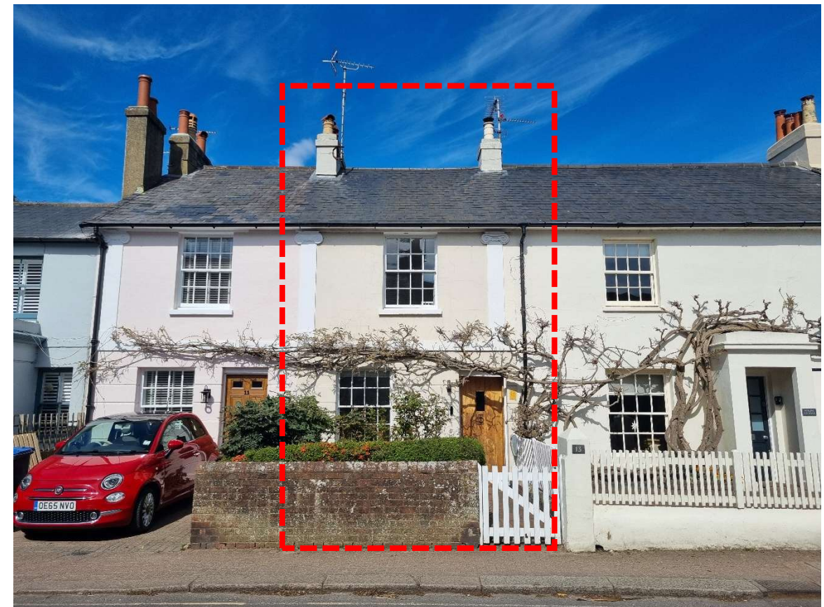
Above: Existing south facing street elevation
