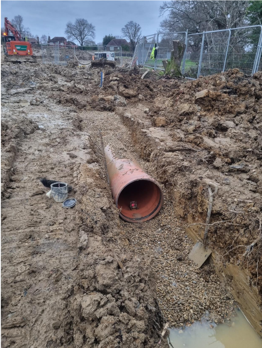
Photo 57 – Pipe between manholes S38-S36
