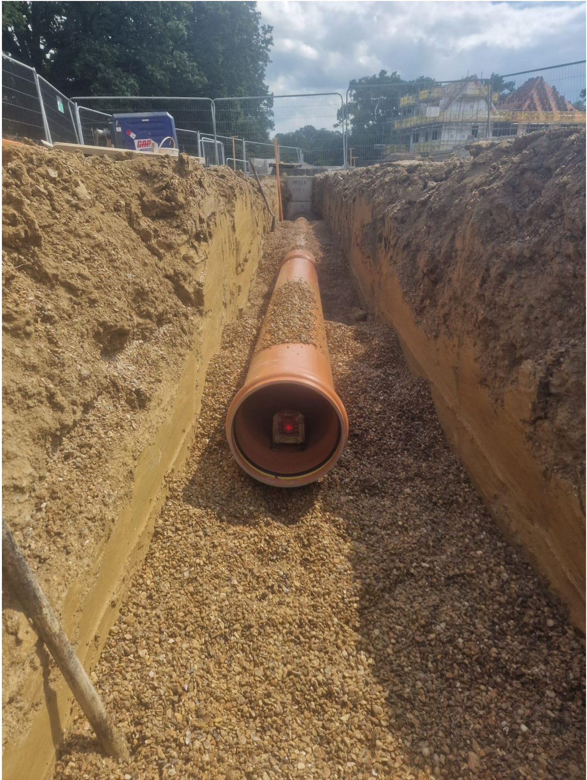
Photo 50 – Pipe between manholes S34-S33
