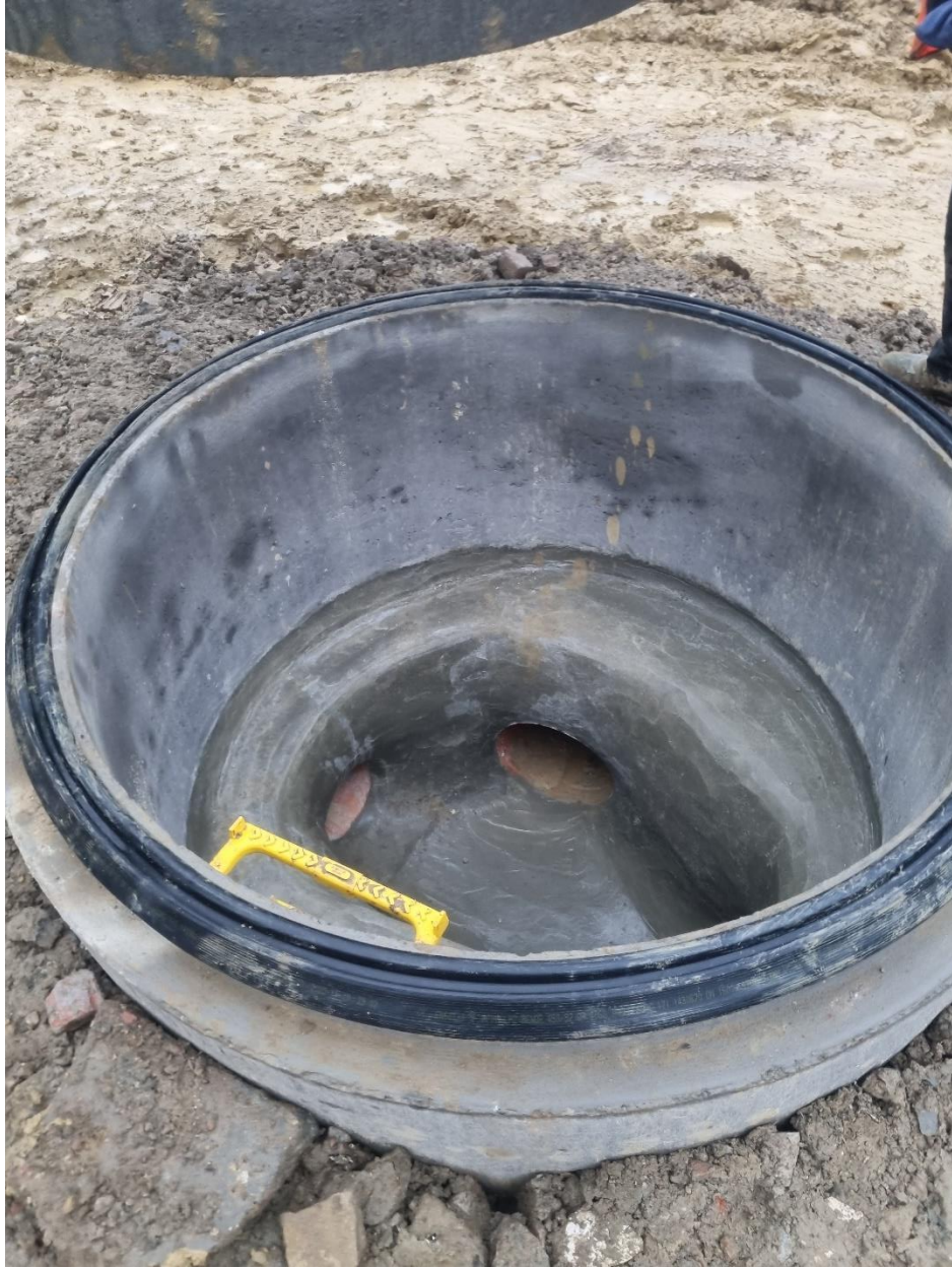
Photo 25 – Base of manhole S28
