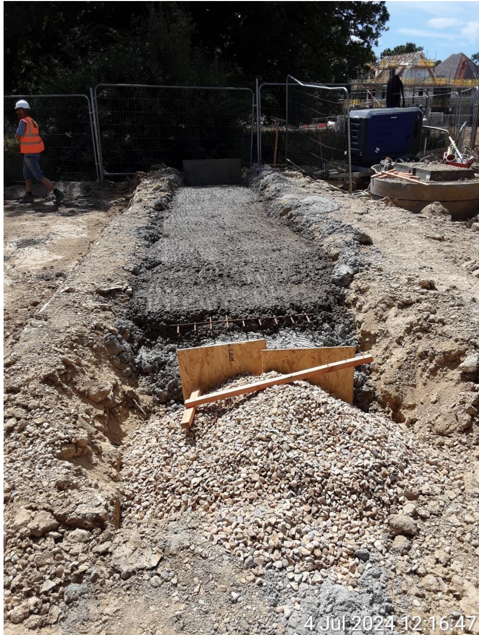
Photo 20 – Culvert B installation
