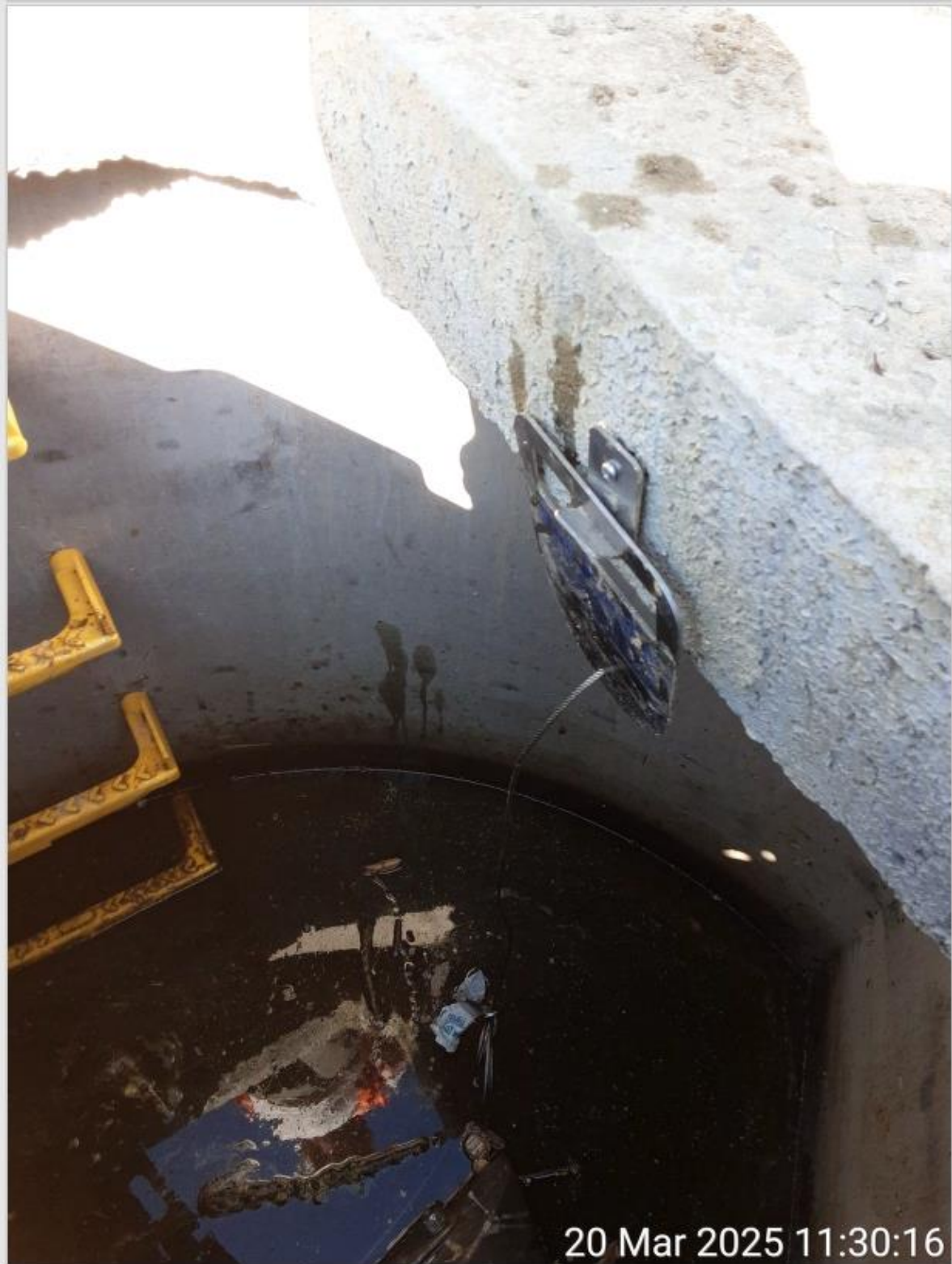
Photo 11 – Hydro-brake pull handle
