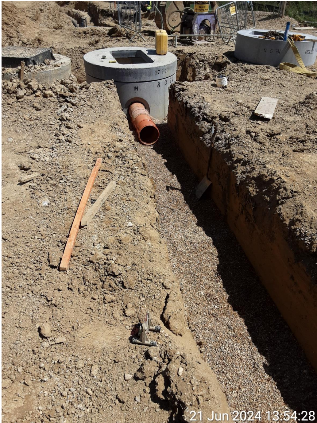
Photo 47 – Pipe between manholes S33-S32
