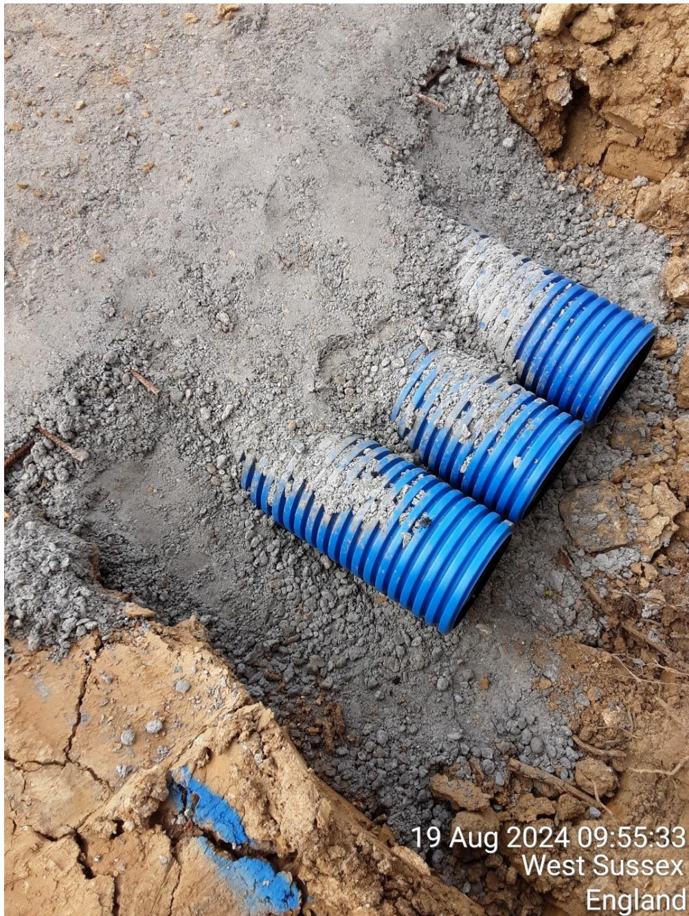
Photo 23 – Culvert C installation
