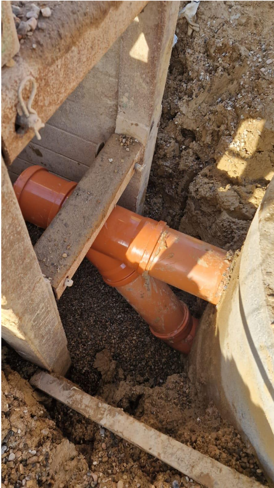
Photo 36 – Backdrop to manhole S24
