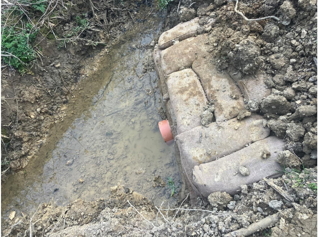
Photo 14 – View of outfall
