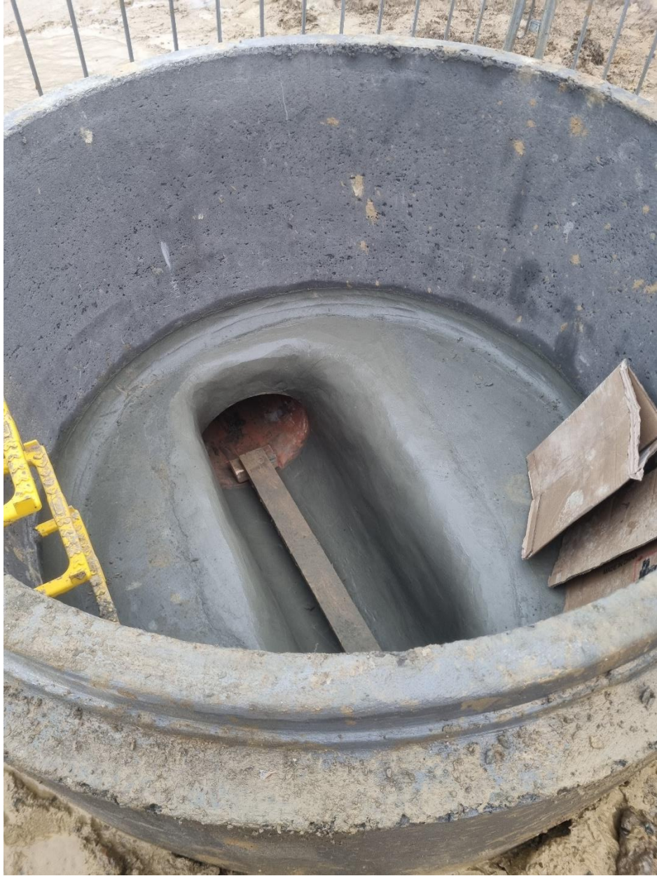
Photo 26 – Base of manhole S29
