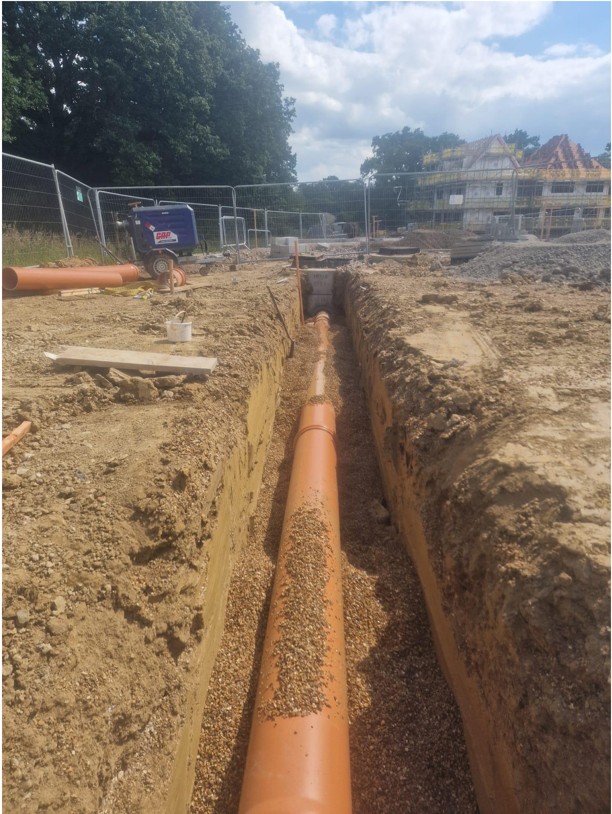
Photo 49 – Pipe between manholes S34-S33
