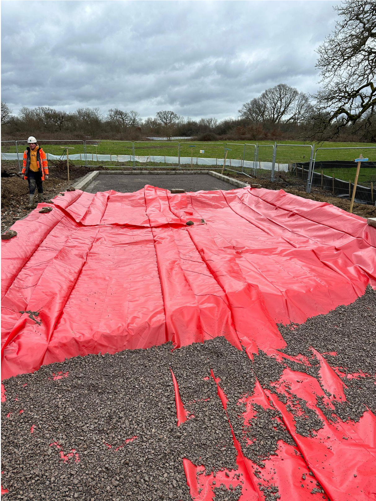
Photo 18 – Culvert A membrane installation
