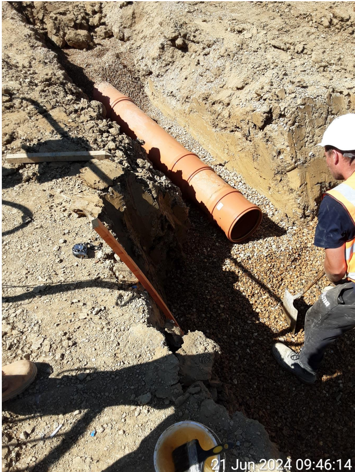
Photo 46 – Pipe between manholes S33-S32
