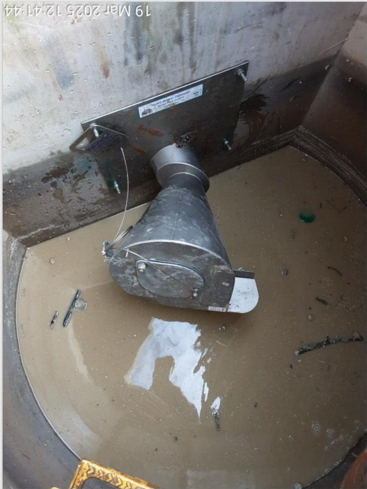
Photo 10 – Hydro-brake installed
