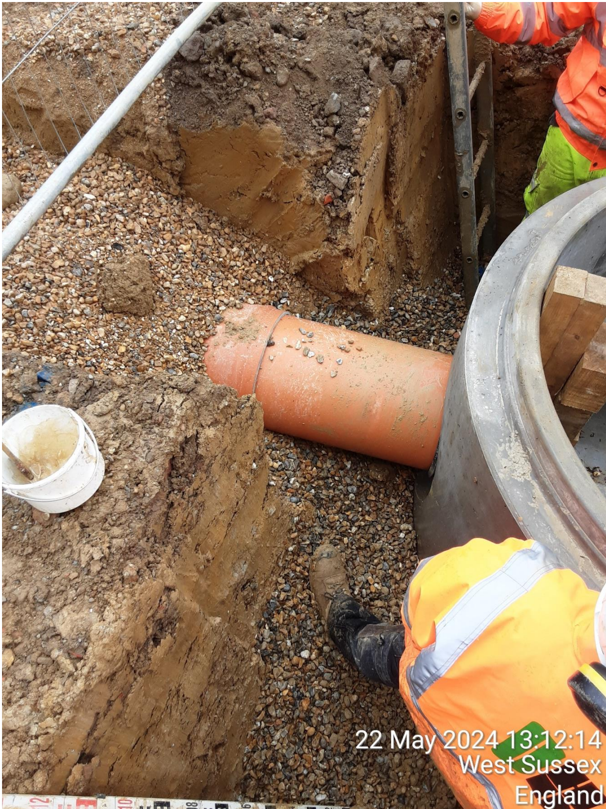
Photo 52 – Pipe between manholes S35-S34
