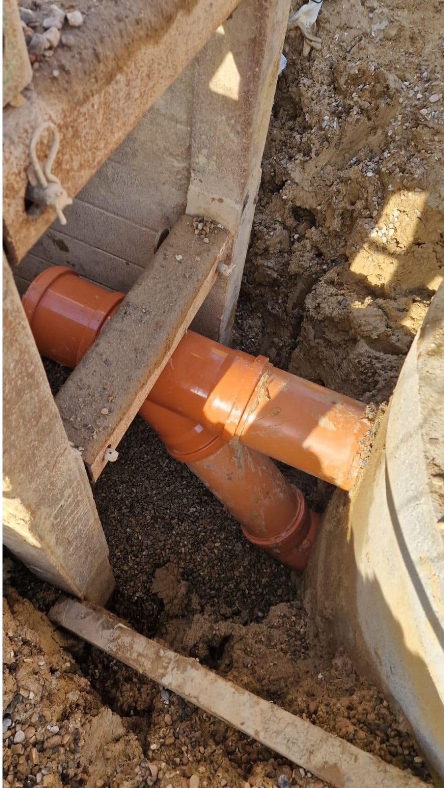
Photo 24 – Back drop to manhole S24
