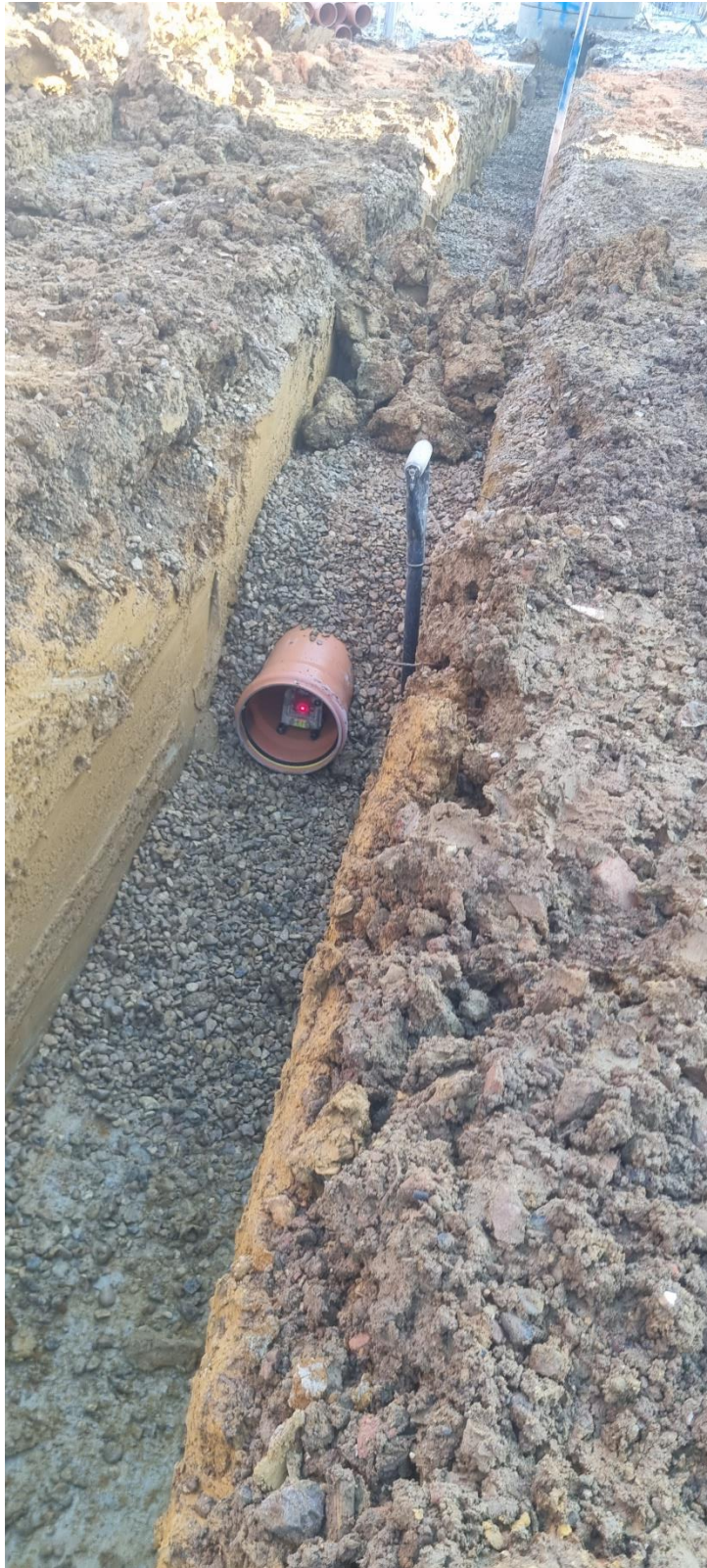
Photo 40 – Pipe between manholes S28-S27
