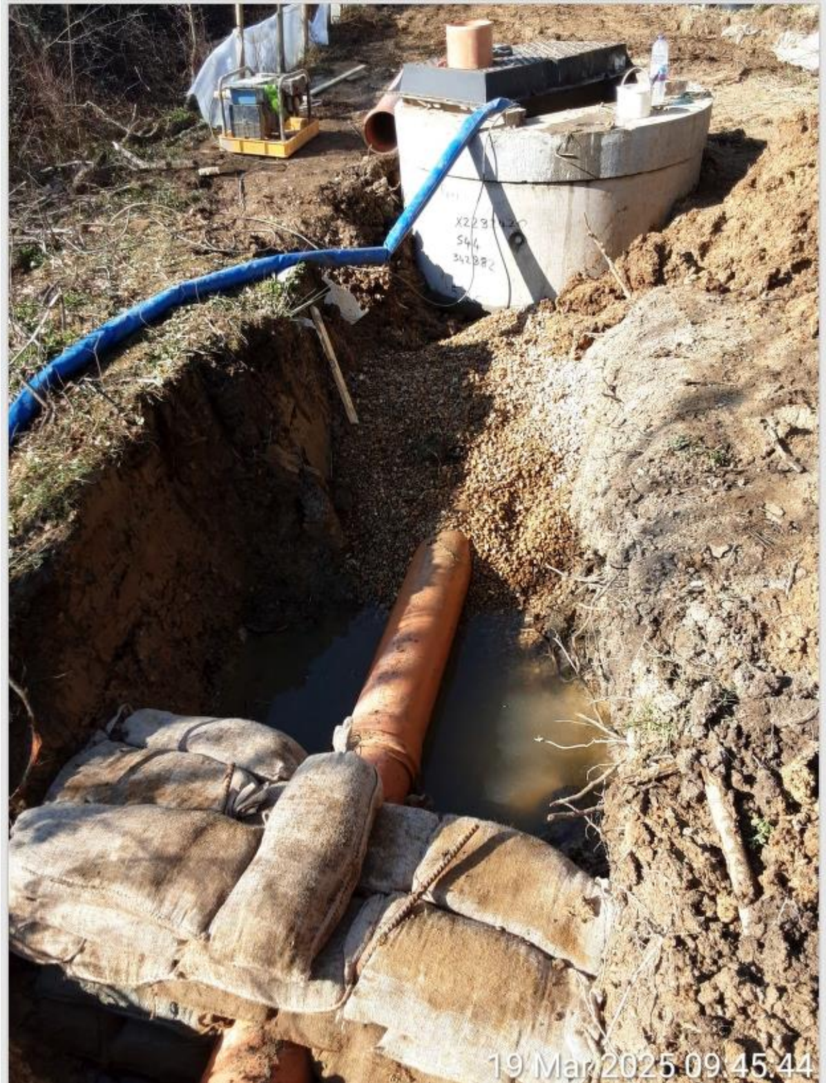
Photo 13 – View of manhole S44 and outfall
