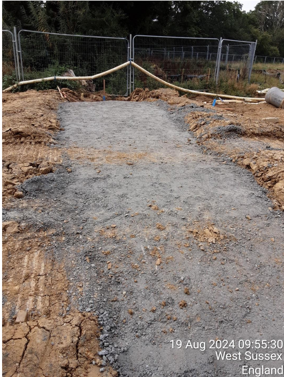
Photo 22 – Culvert C installation
