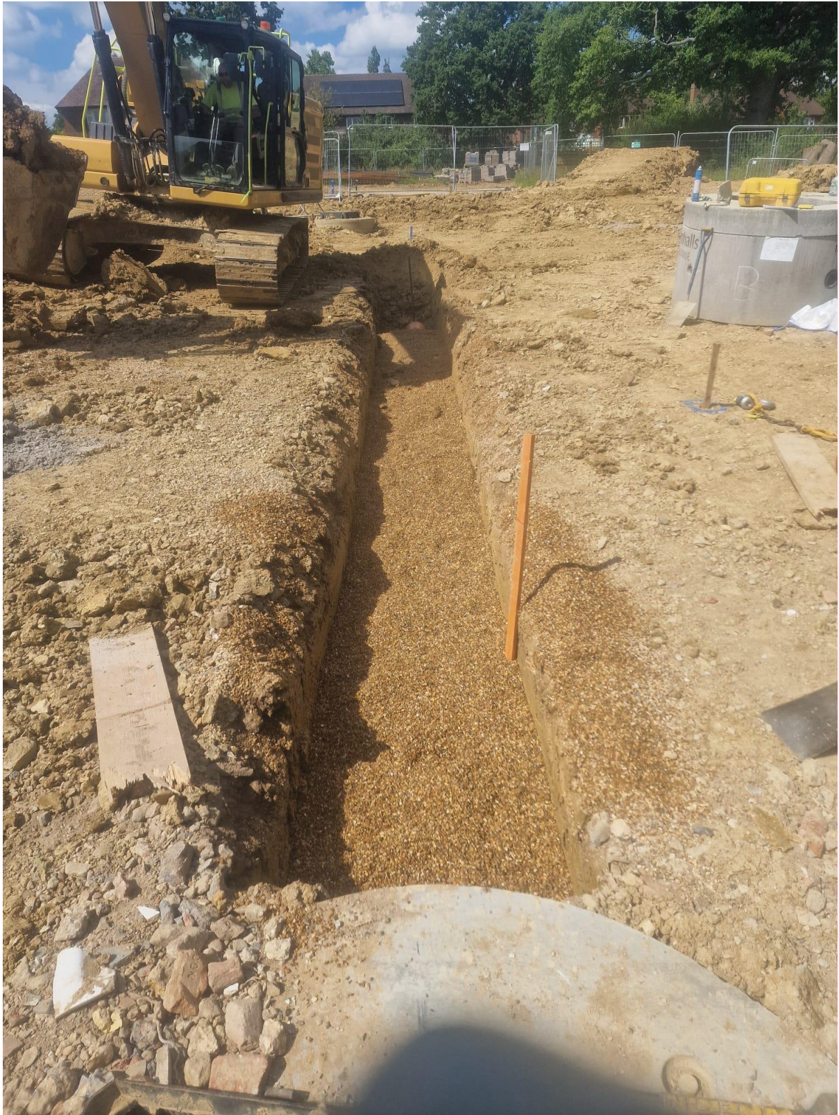
Photo 51 – Pipe between manholes S34-S33
