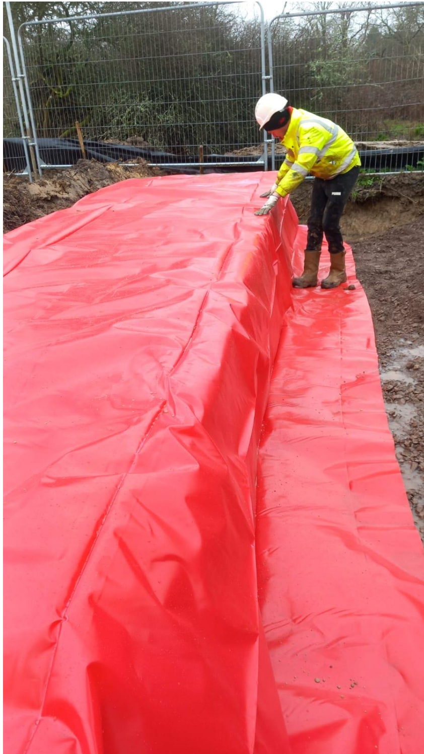
Photo 16 – Culvert A membrane installation
