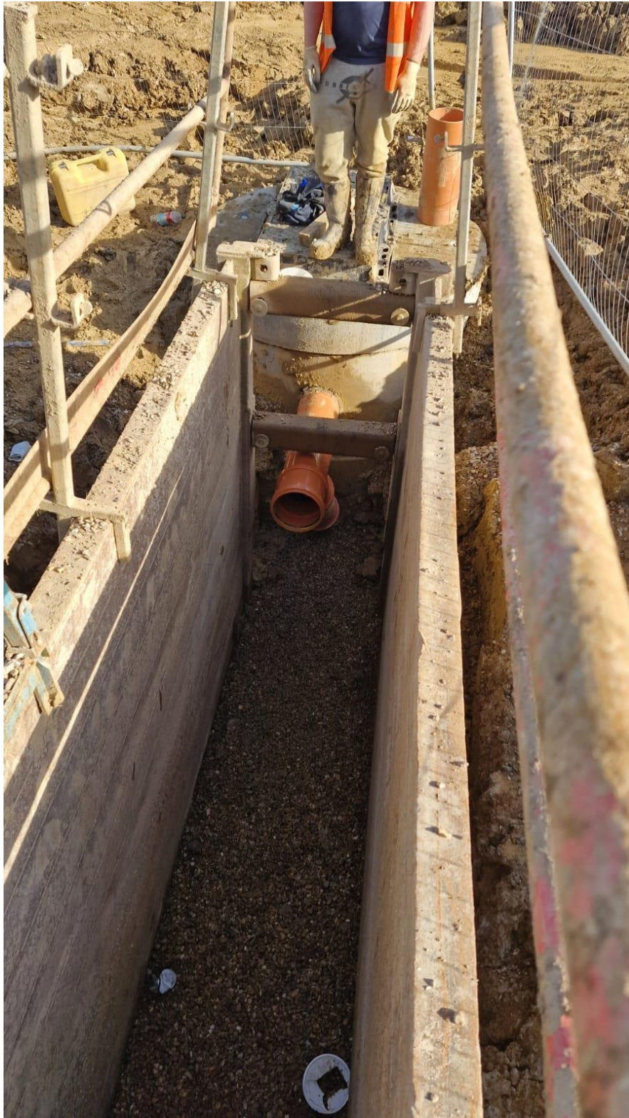
Photo 38 – Pipe between manholes S23-S24
