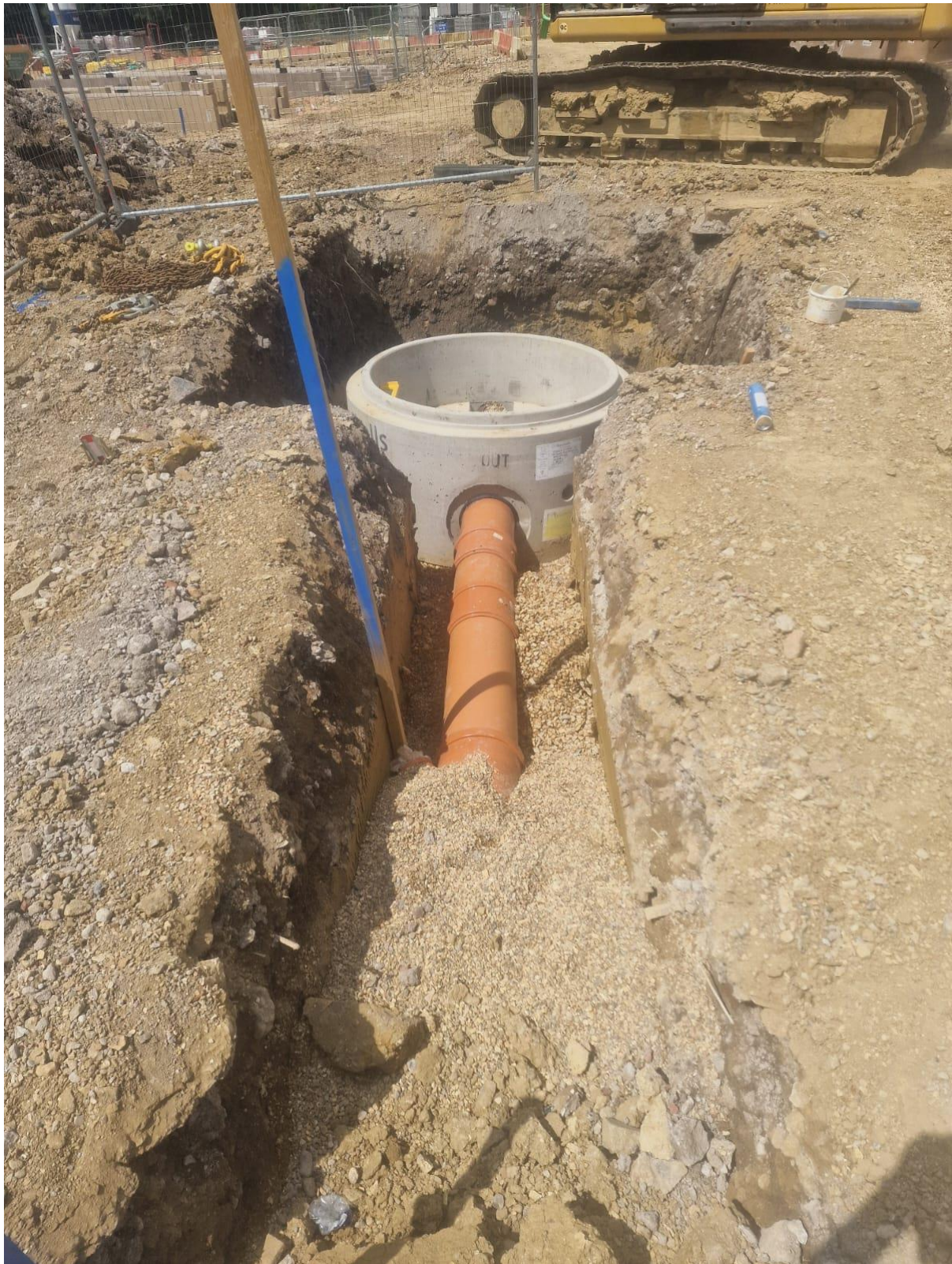
Photo 45 – Pipe between manholes S33-S32
