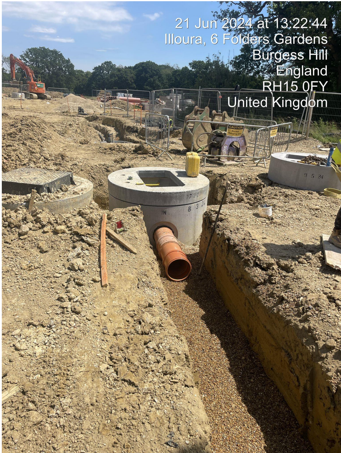
Photo 44 – Pipe between manholes S32-S33
