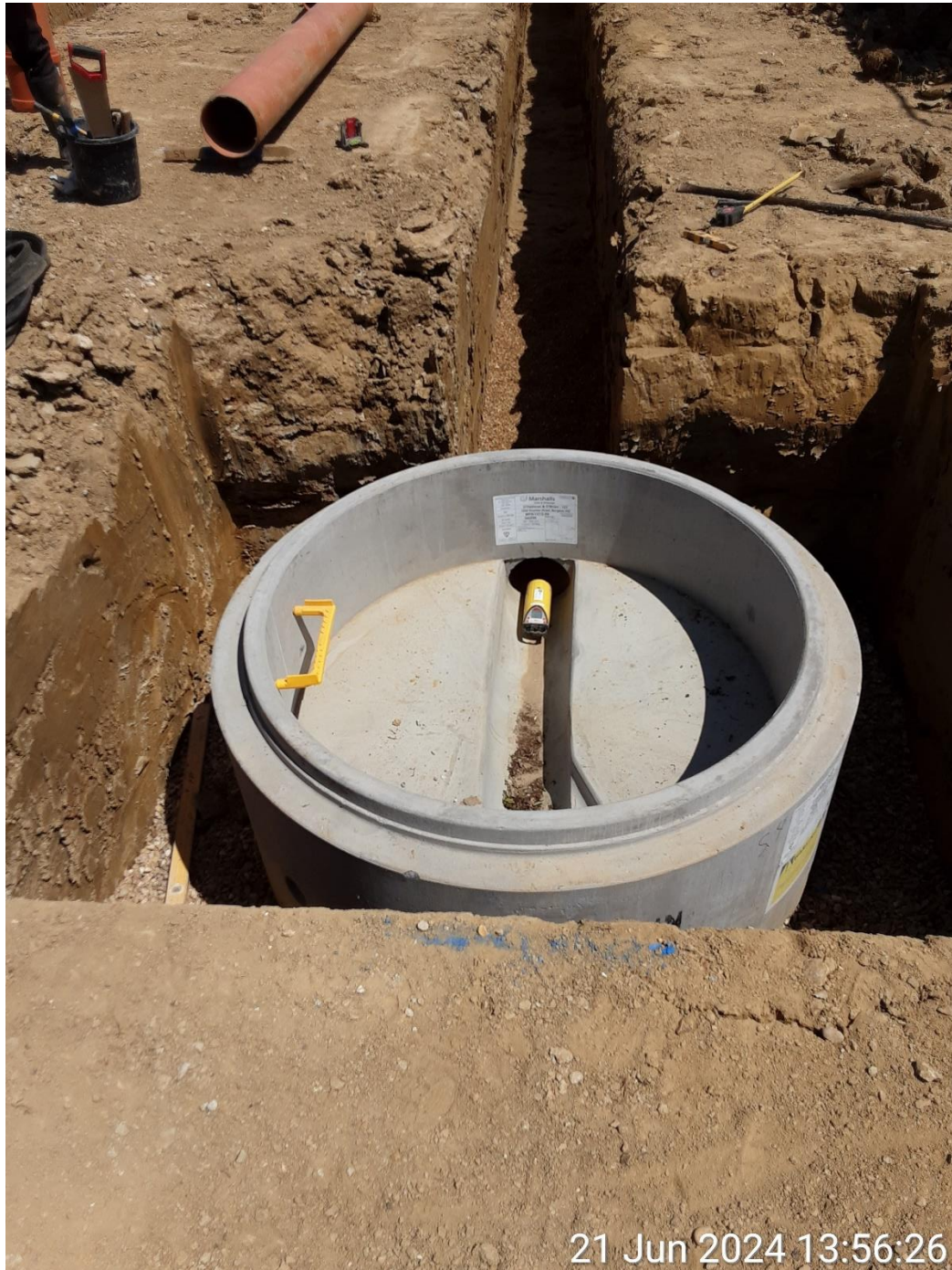
Photo 48 – Pipe between manholes S33-S32
