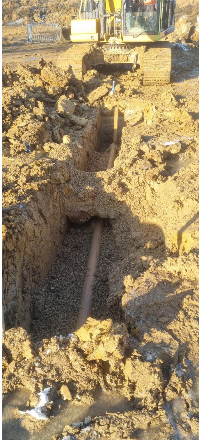
Photo 56 – Pipe between manholes S36-S35
