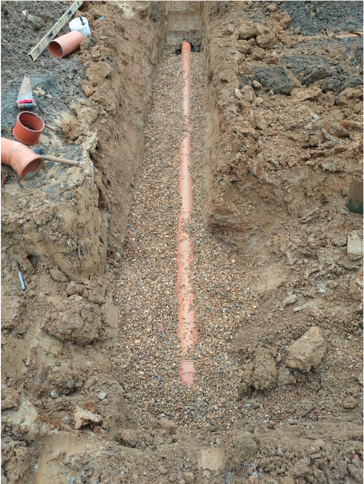
Photo 39 – Pipe between manholes S23-S24
