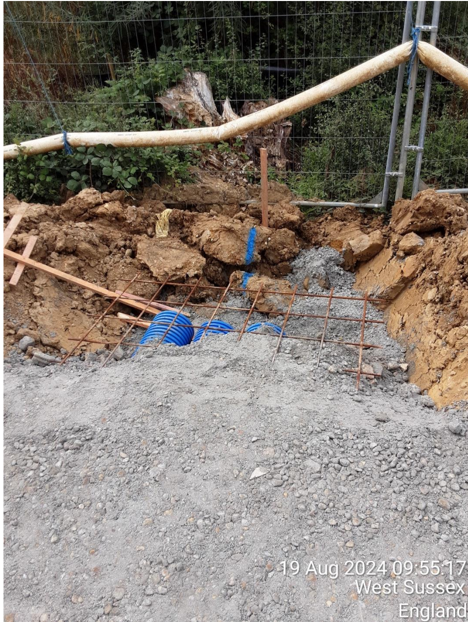
Photo 21 – Culvert C installation
