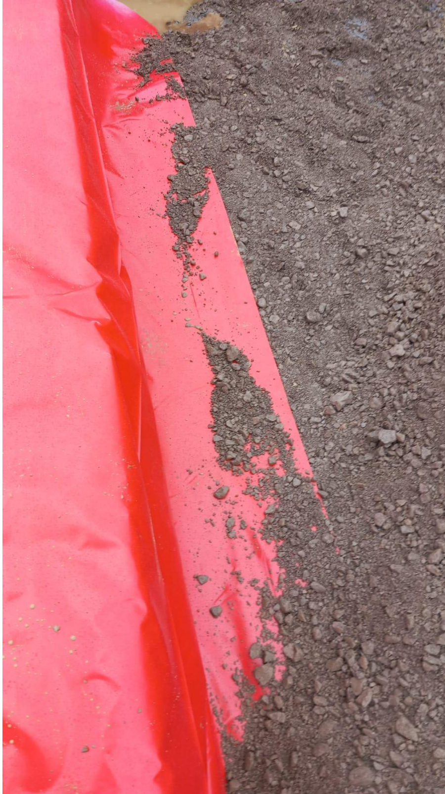
Photo 17 – Culvert A membrane installation
