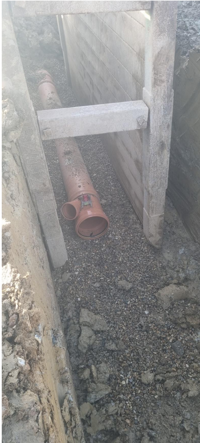
Photo 34 – Pipe between manholes S22-S24
