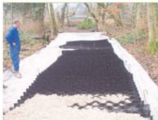
CellWeb during installation.
