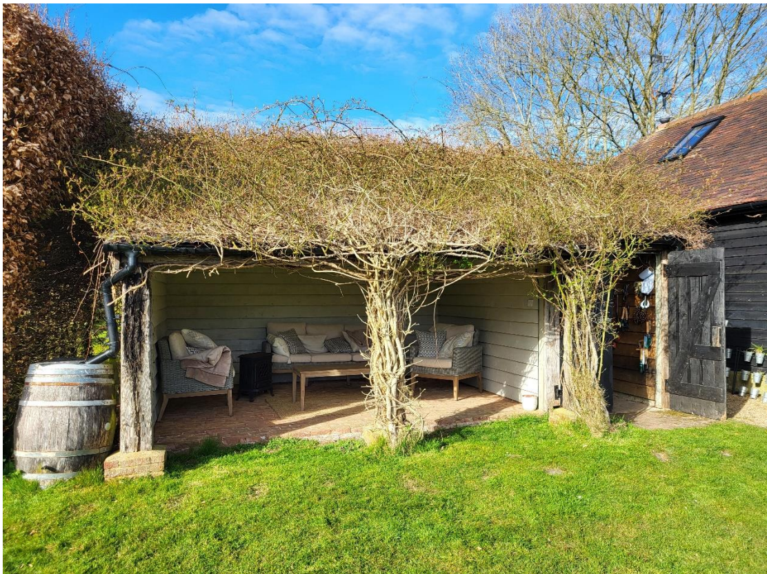
Whilst fabricated from older material, the structure is modern and was probably assembled when the garage was built.
