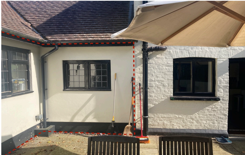
The walls of the existing extension to be removed to allow the building to be extended westwards.
