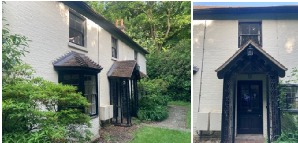
The polite western elevation with its decorative porch and sash windows.
