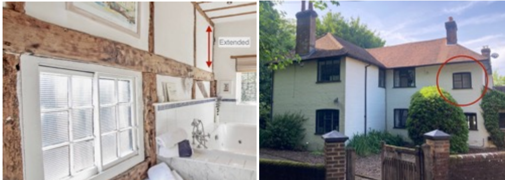
The extended timber-frame in the bathroom and window set low, well below the eaves.
