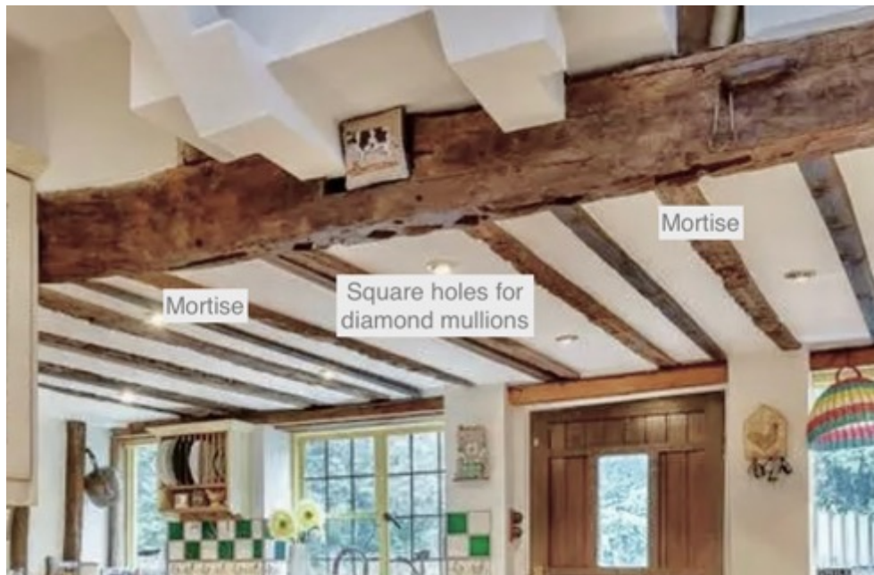
The beam in the kitchen containing evidence of a former window.
