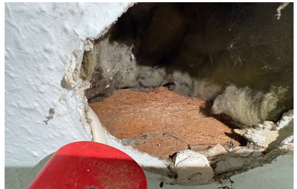
Small opening confirming the presence of modern finishing covering the roof structure.
