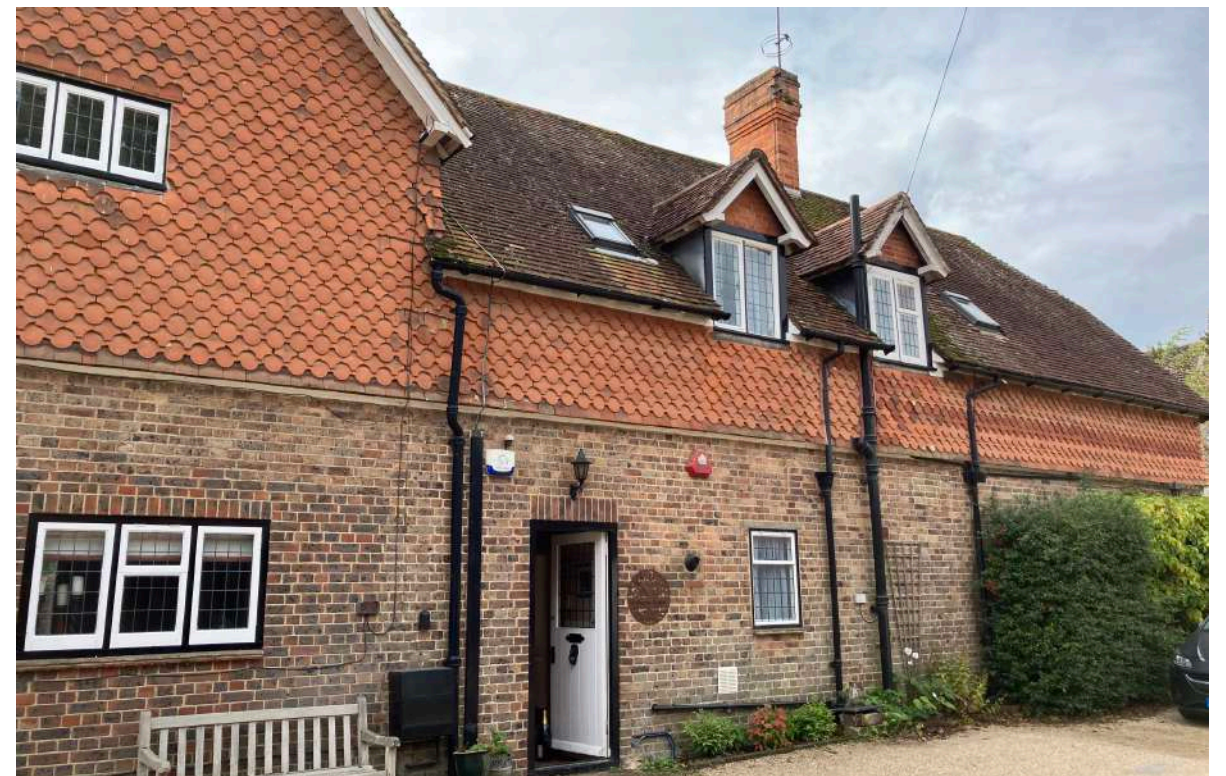
North elevation of Mulberry Cottage
