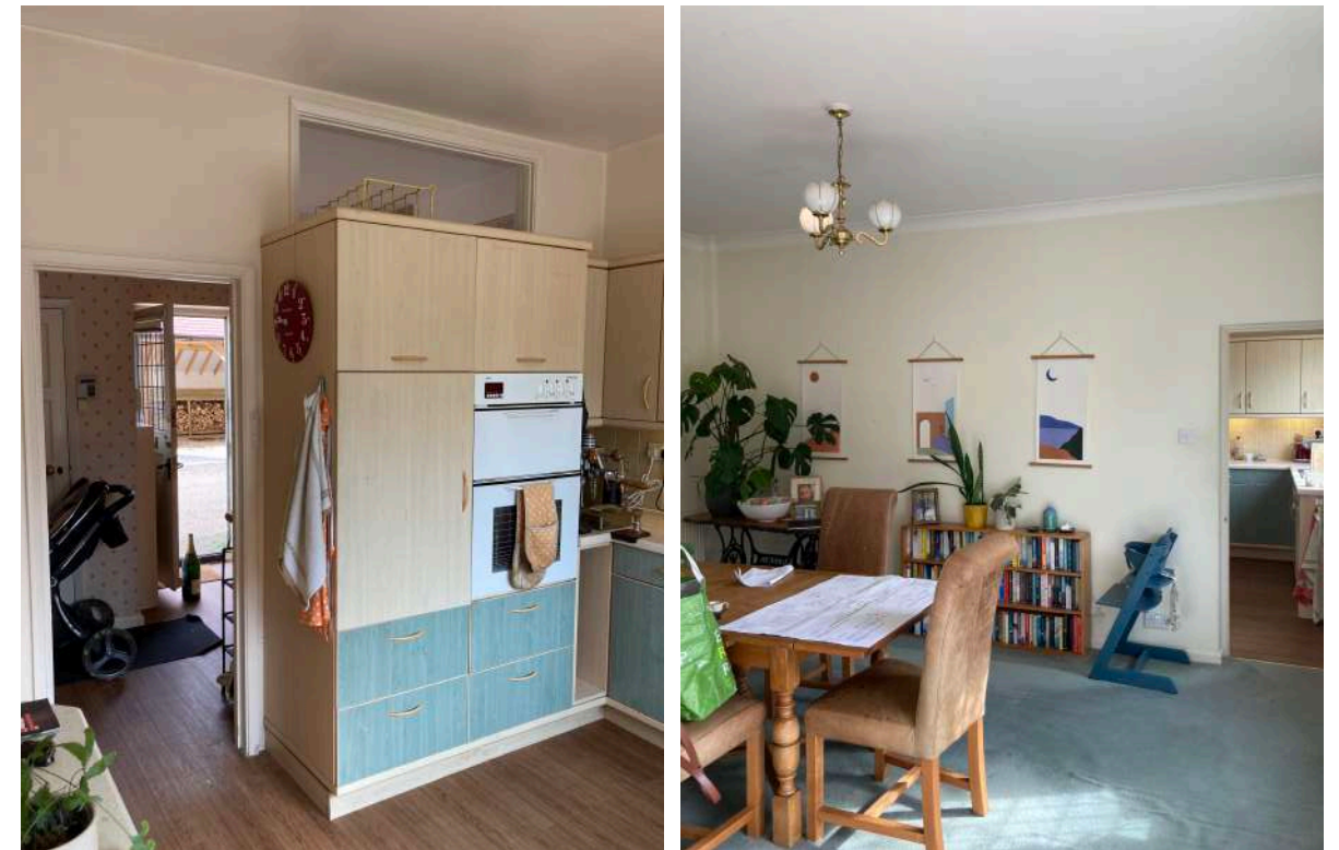
Example of modern partitions to be removed.
