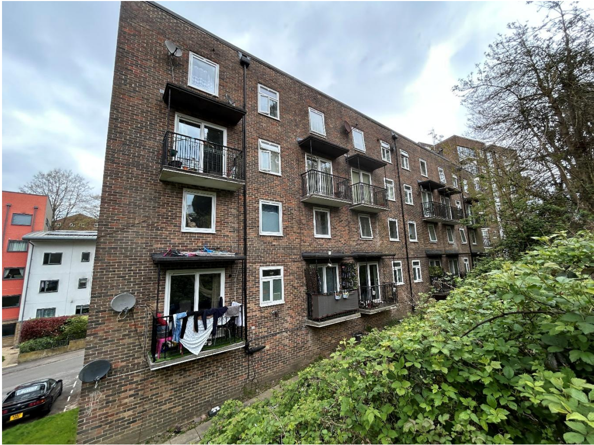
Existing Private balconies.
