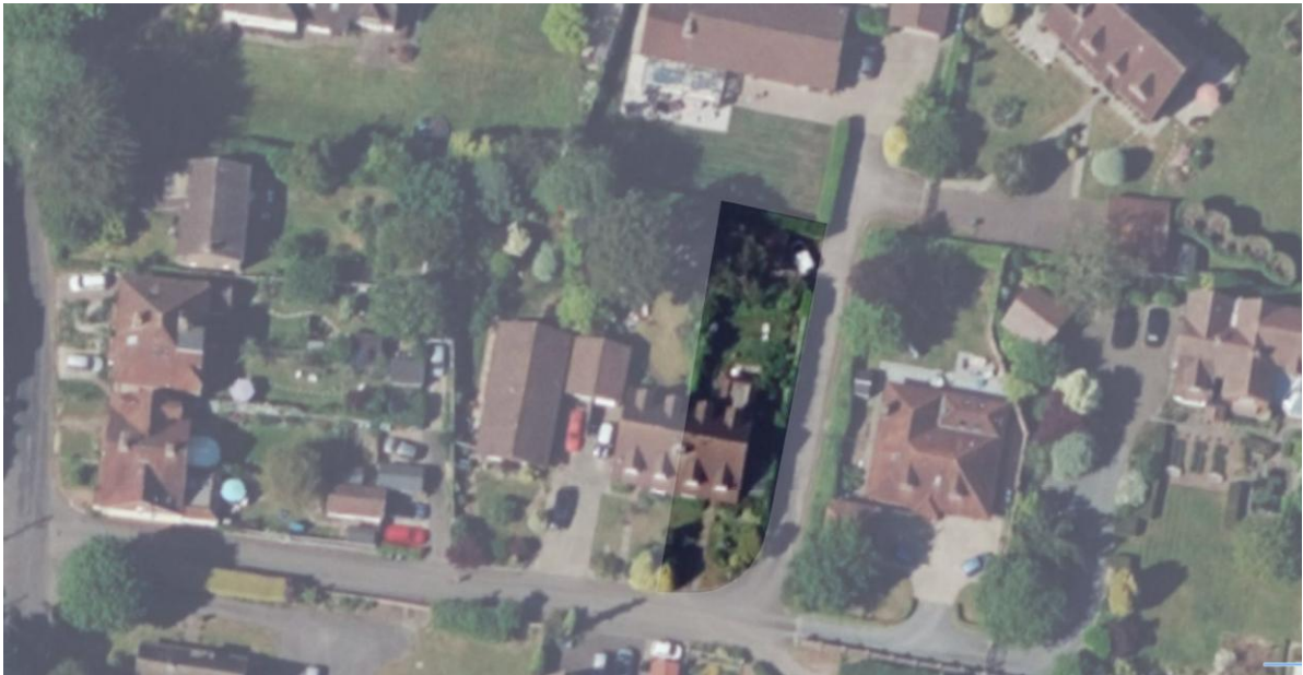
Existing aerial View of 41 College Lane
