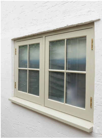
Salisbury Joinery Conservation+
