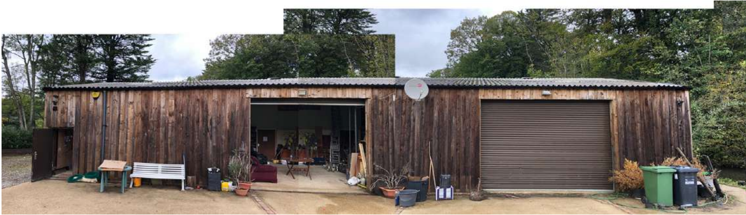
E01 - Looking North west (front elevation of timber clad barn)
