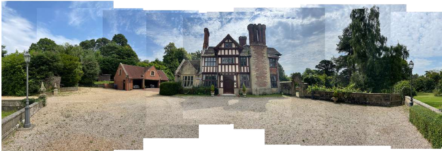
B01 - Looking South East towards Chownes Mead with garages to left of frame
