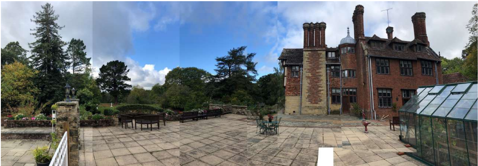
C04 - Looking North West towards Chownes Mead and terrace
