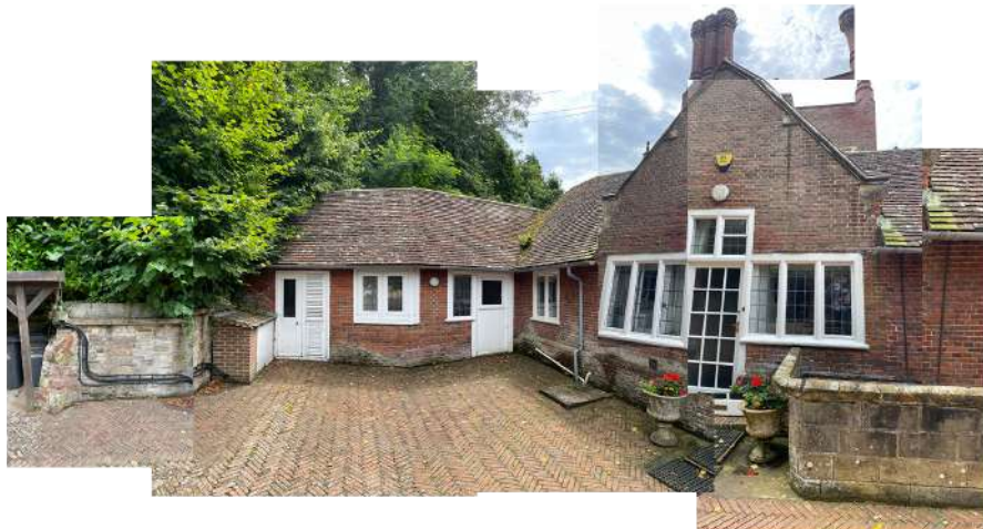
B04 - Rear of Chownes Mead looking South
