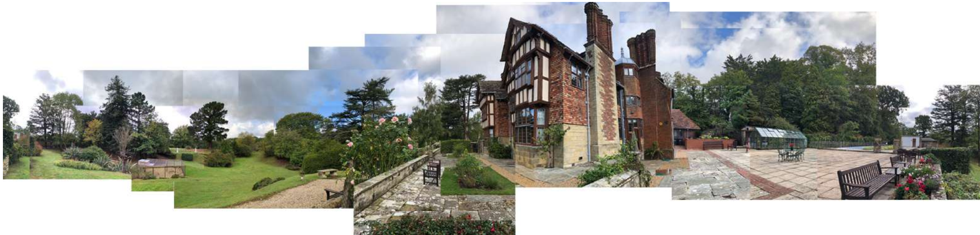
B06 - Looking North towards Chownes Mead, terraces and gardens
