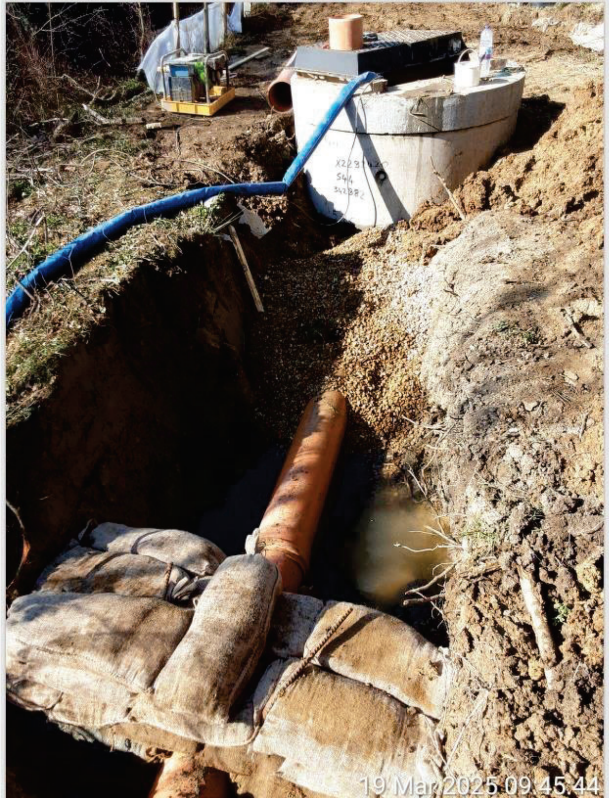
Photo 13 – View of manhole S44 and outfall
