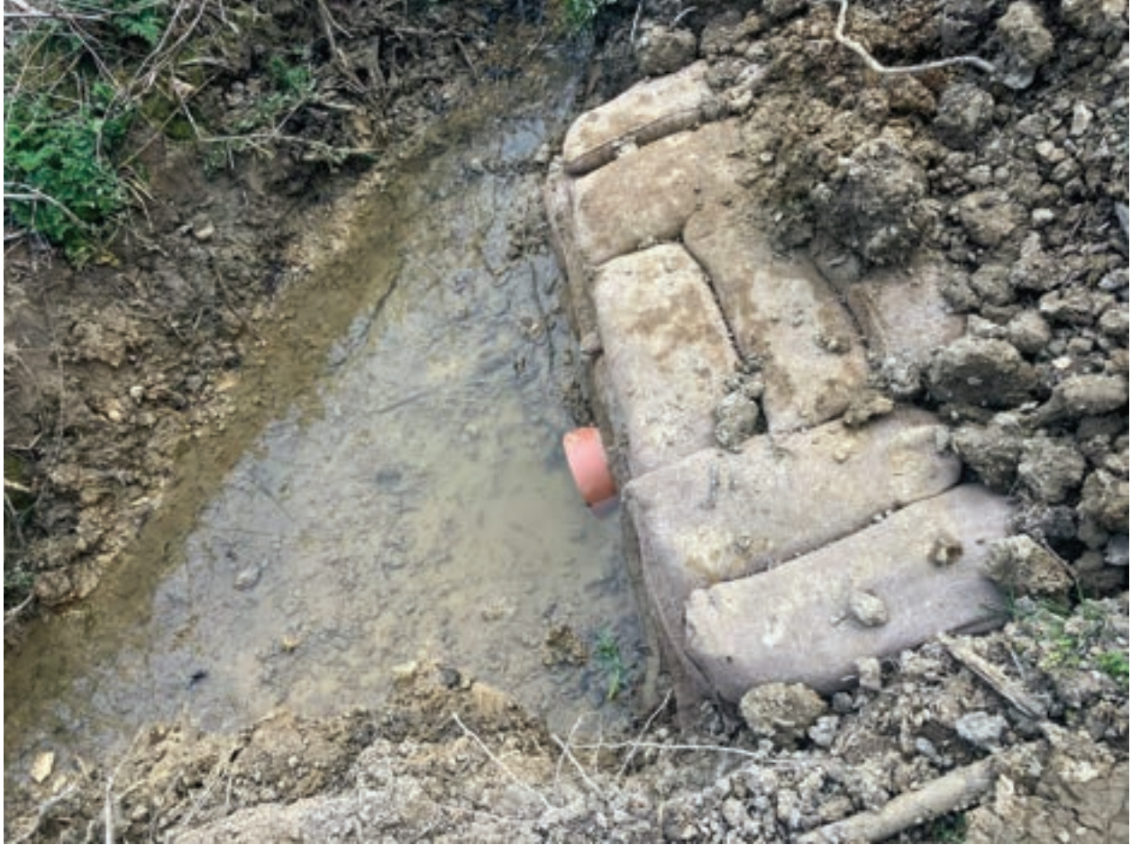
Photo 14 – View of outfall
