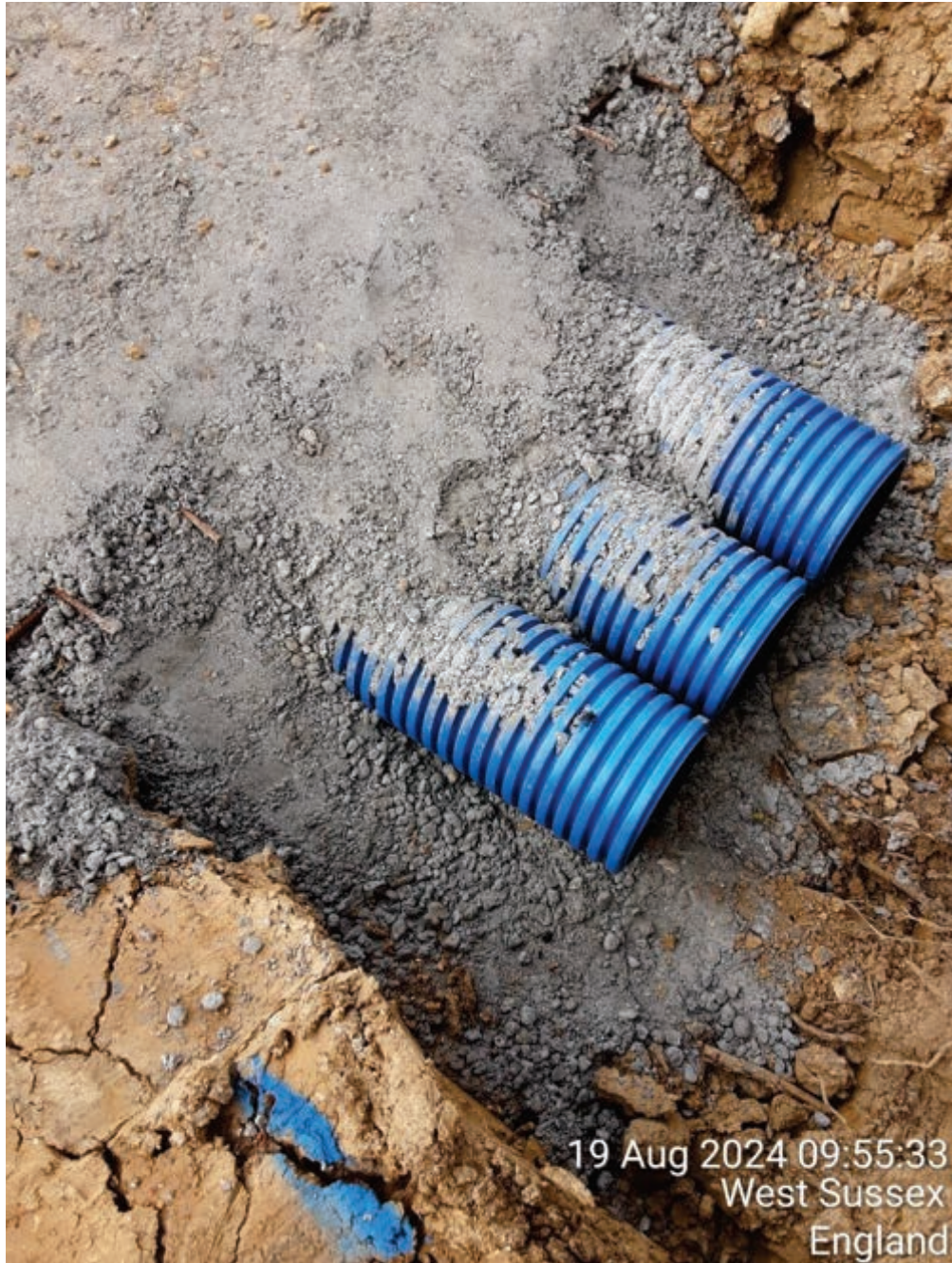
Photo 23 – Culvert C installation
