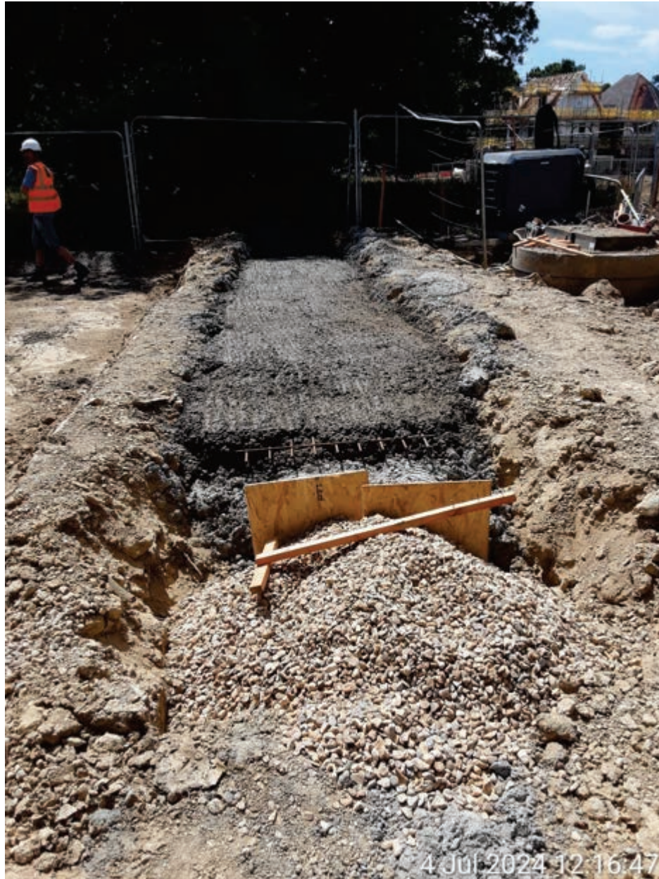
Photo 20 – Culvert B installation
