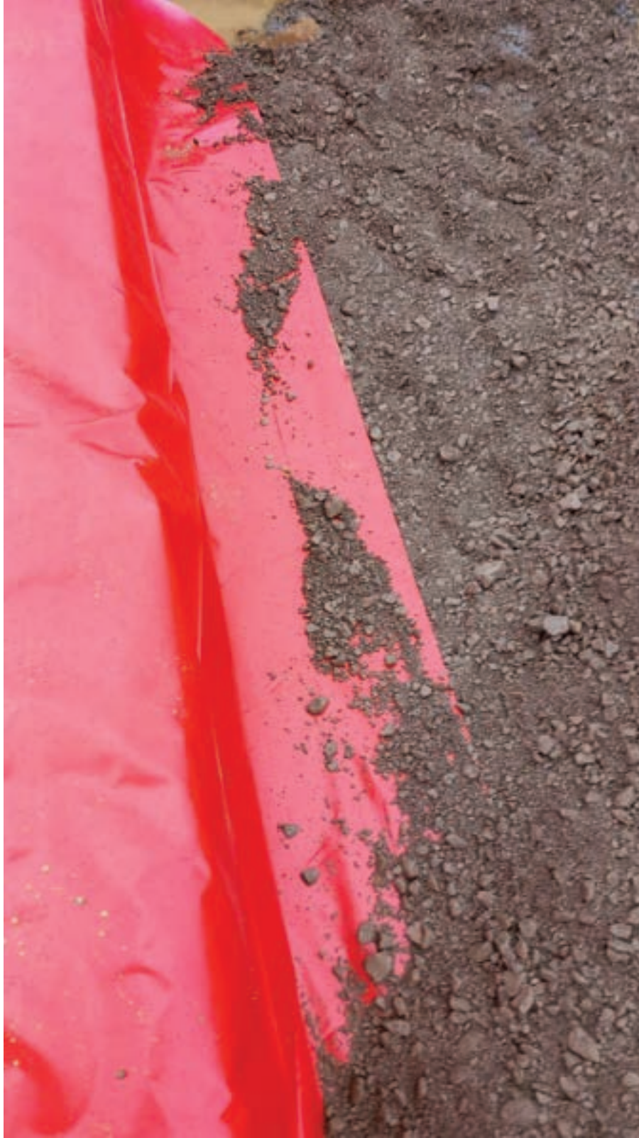
Photo 17 – Culvert A membrane installation
