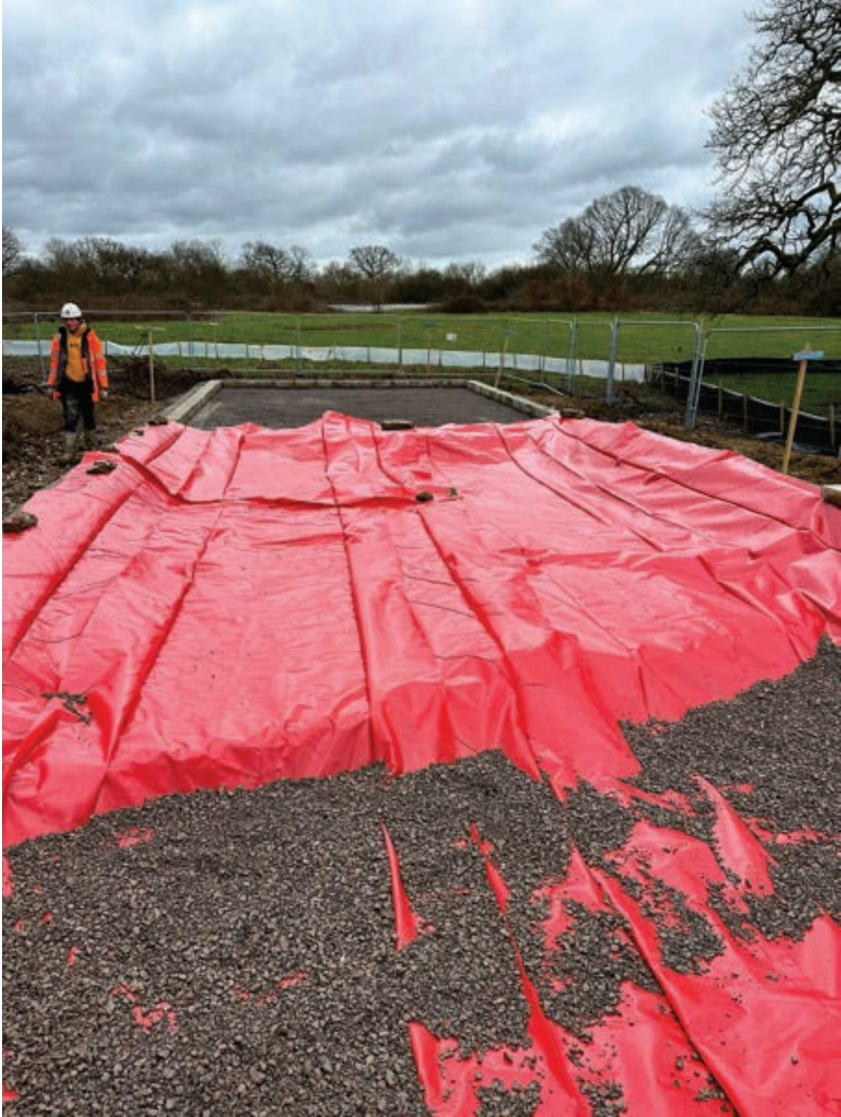
Photo 18 – Culvert A membrane installation
