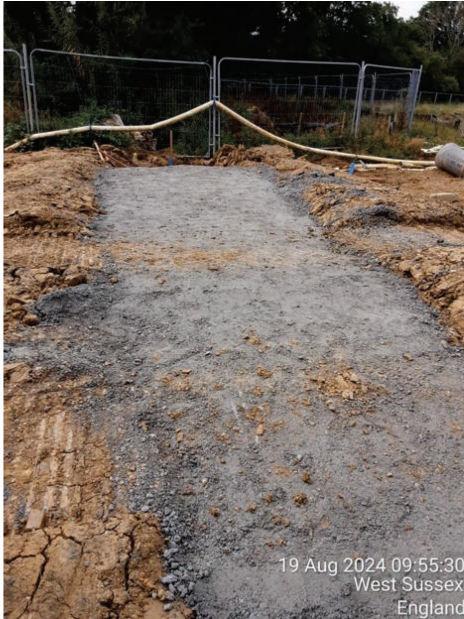
Photo 22 – Culvert C installation
