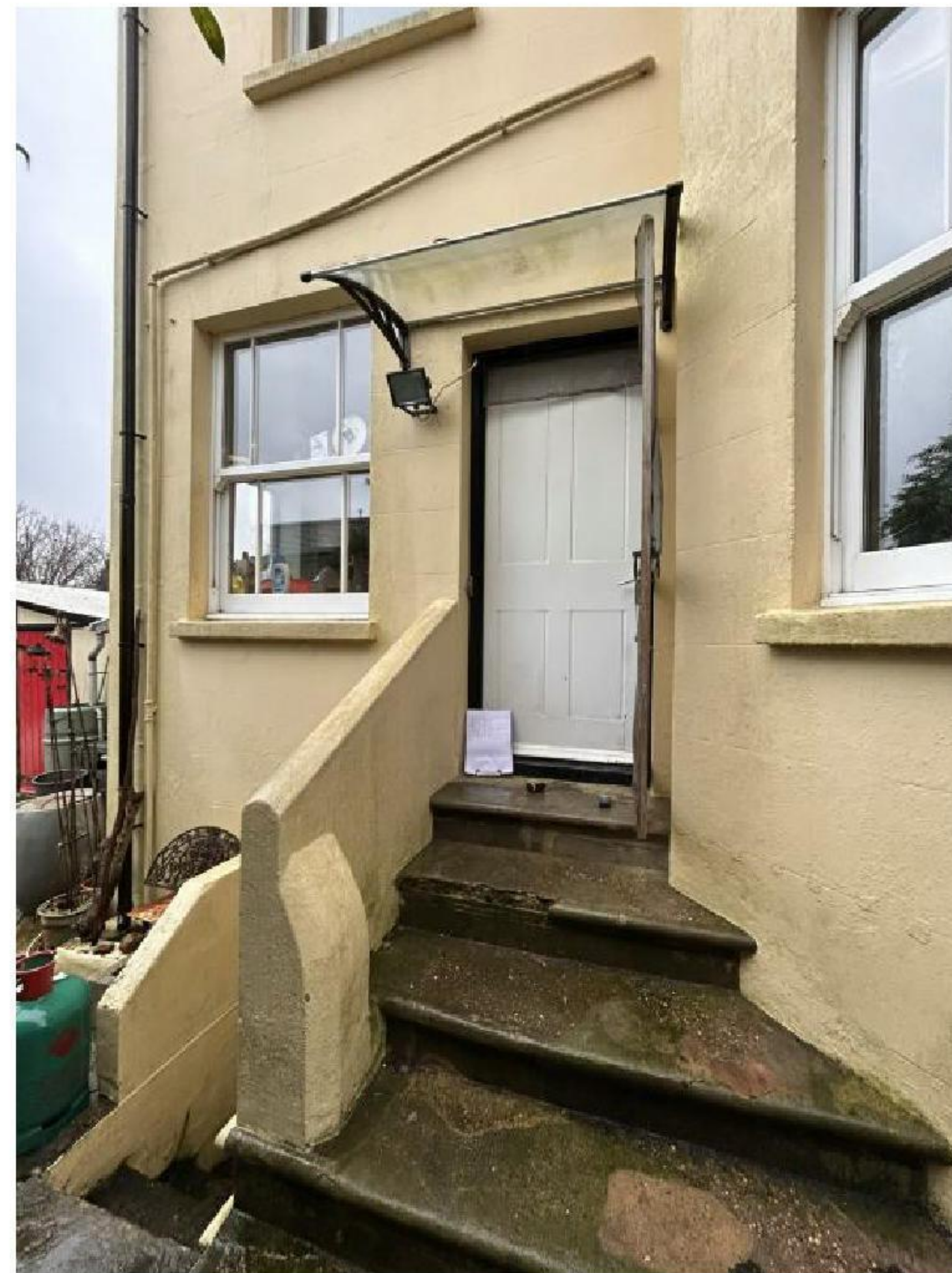
Side view of the rear Kitchen with external steps.
