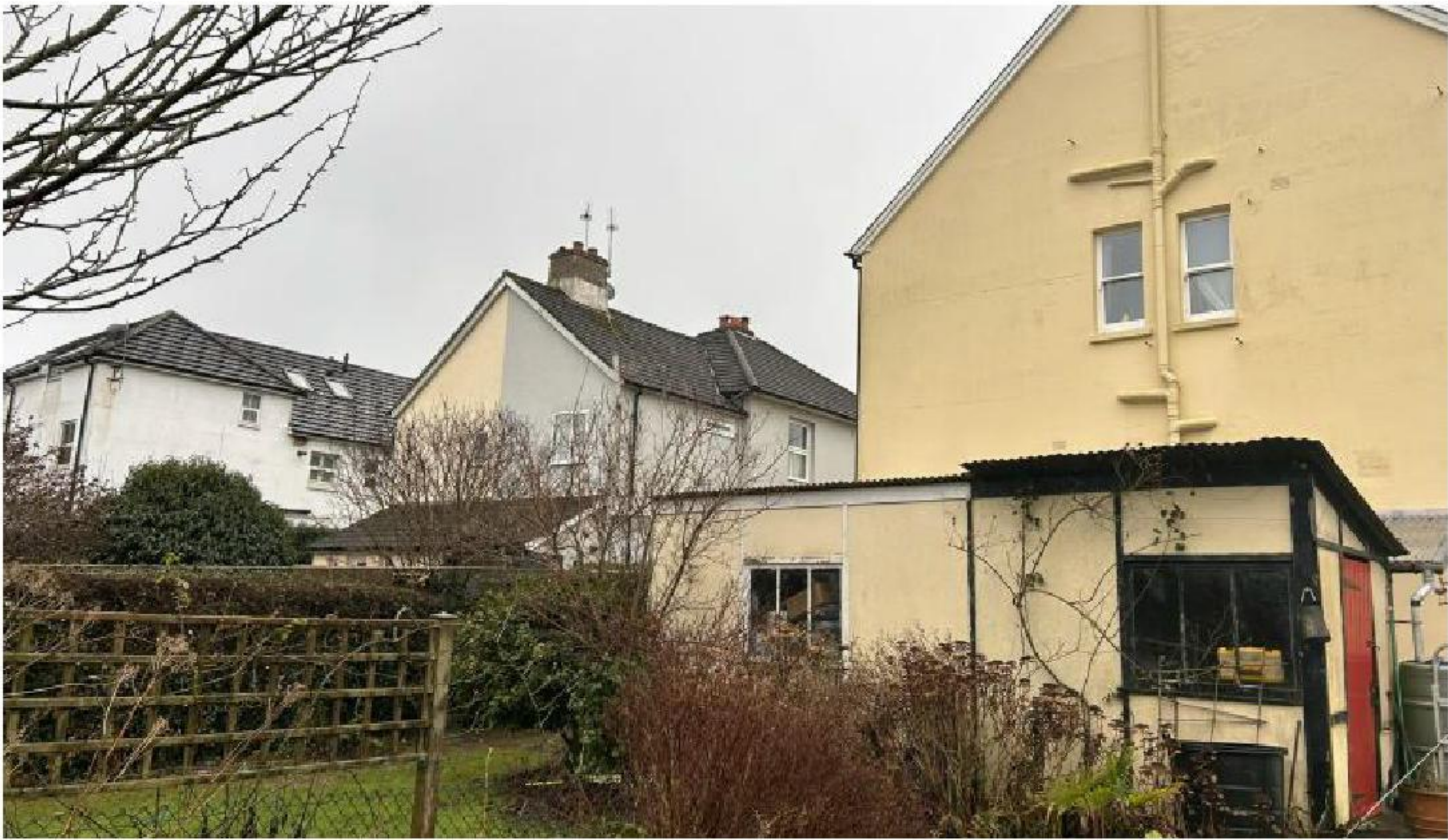
Rear view of No.76 (RHS of image) looking South with semis Nos. 80 & 82 visible beyond.
