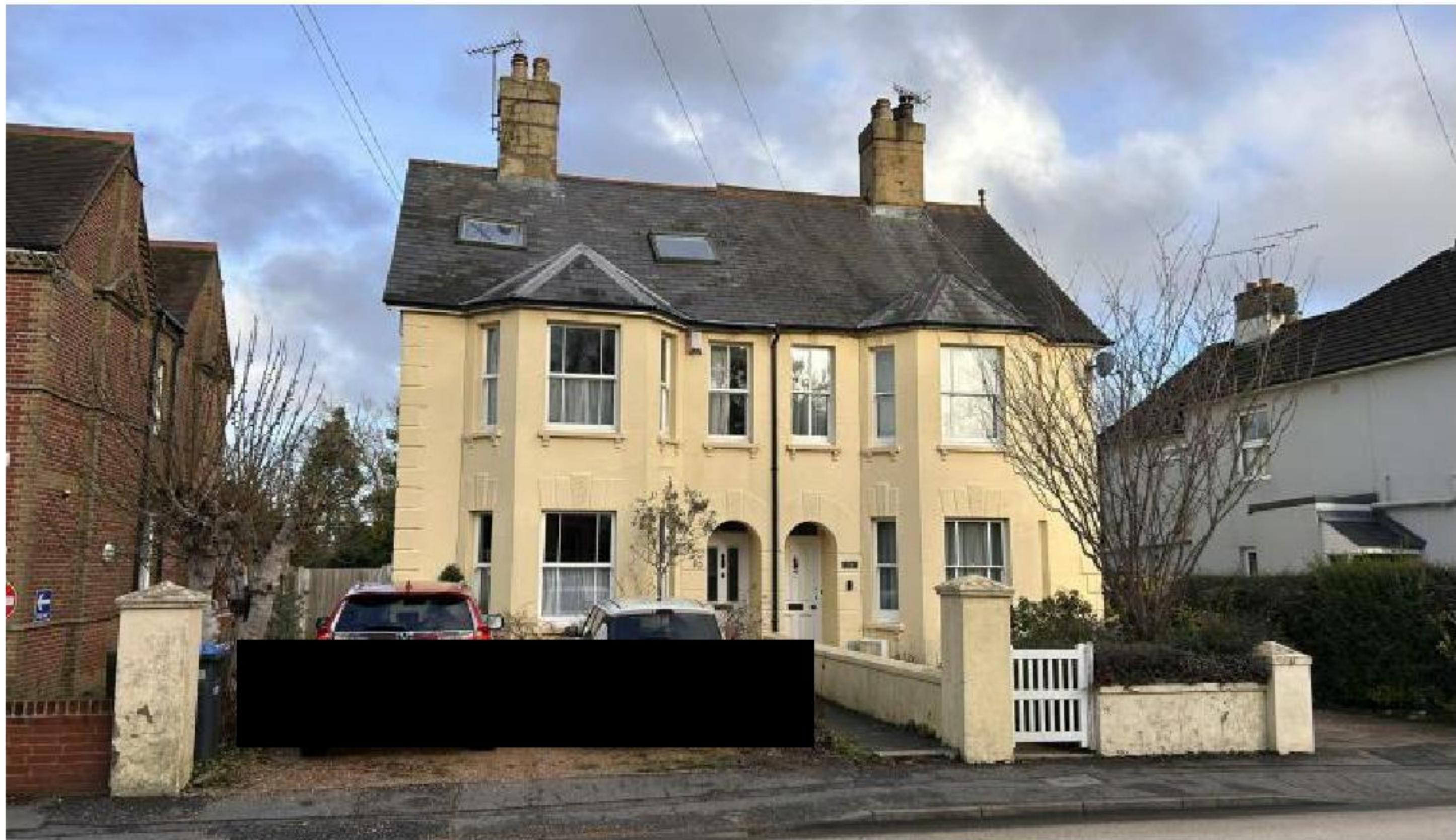
Street View of 76 Moat Road (left hand side of the semi-detached pair). The left hand neighbouring building is a school.
