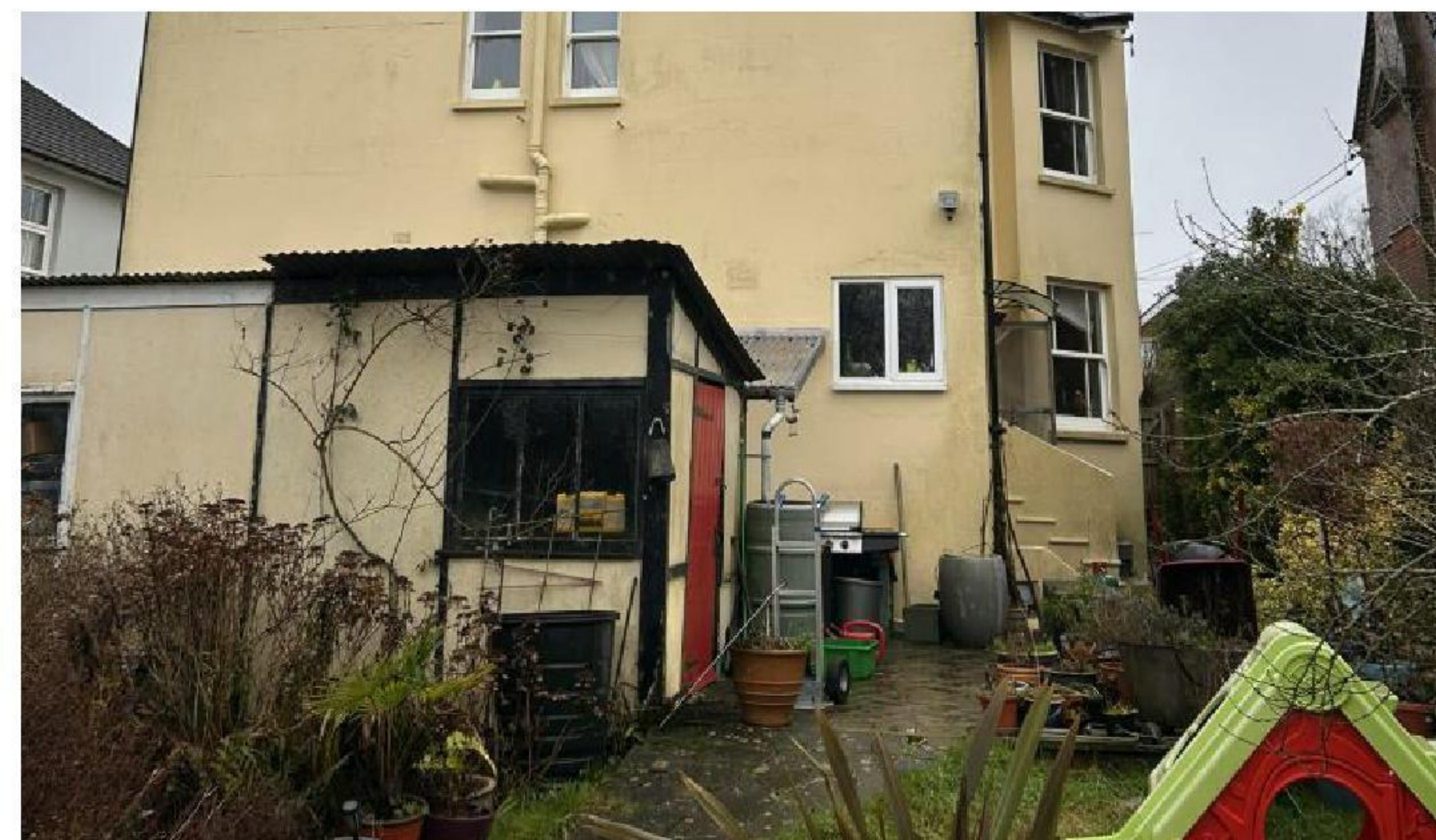
Rear view of the shed and
