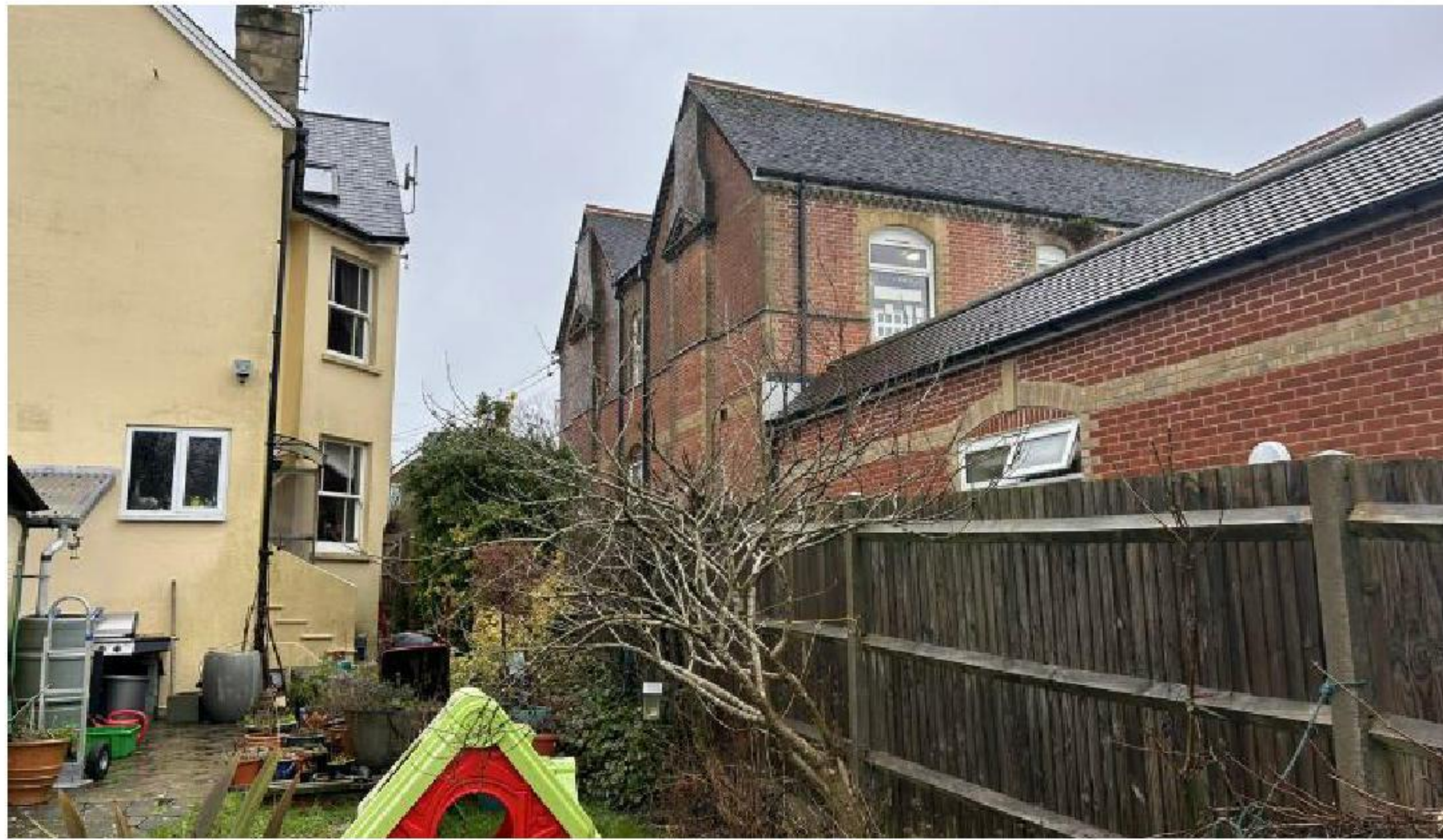
Rear view of No.76 (LHS image) looking West with the school visible on the right of the image.
