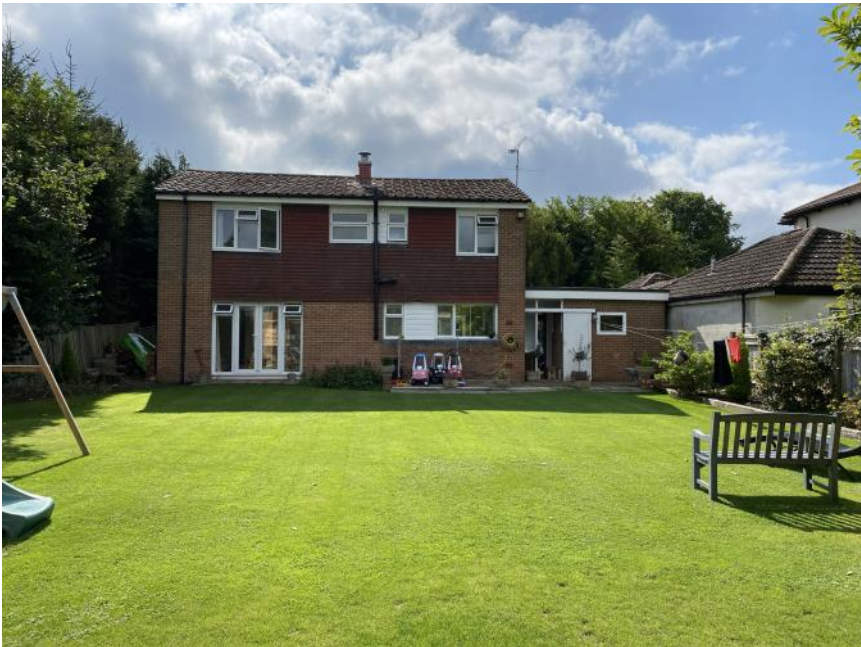
Rear elevation viewed from the garden
