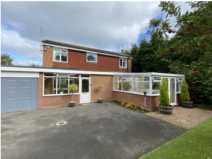
Front elevation viewed from the driveway
