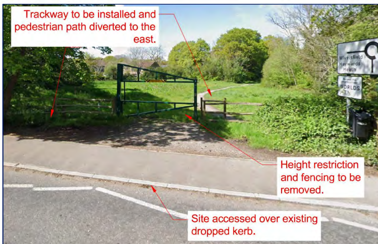
Figure 3.1 – site access location and works.
