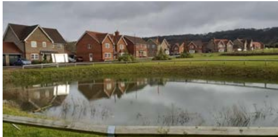
Attenuation basin to manage surface water sustainably
