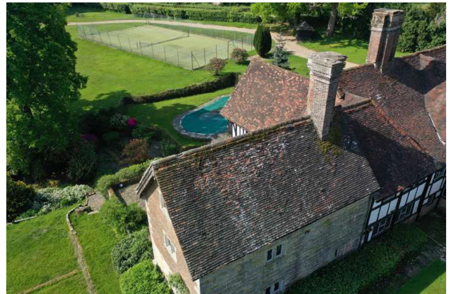
clay plain tile to north slope
