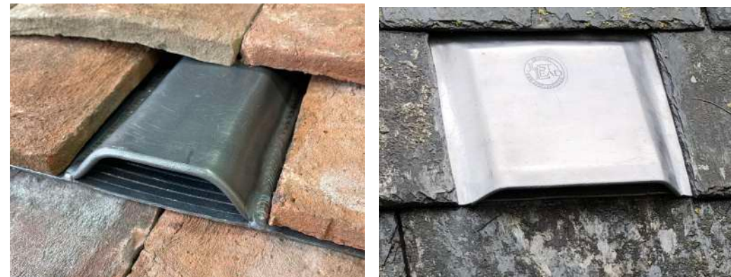
lead bat arch installed in plain clay tile and slate roof
