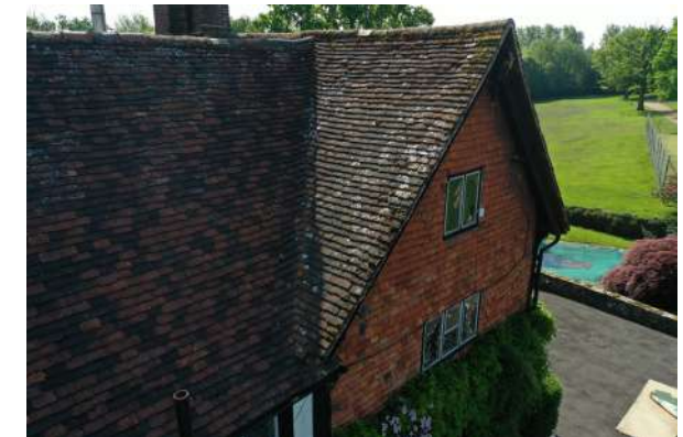
traditional laced tiled valley to west slope adjoining C17th range
