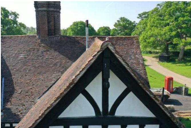
traditional mortar bedded verge with tiled undercloak
