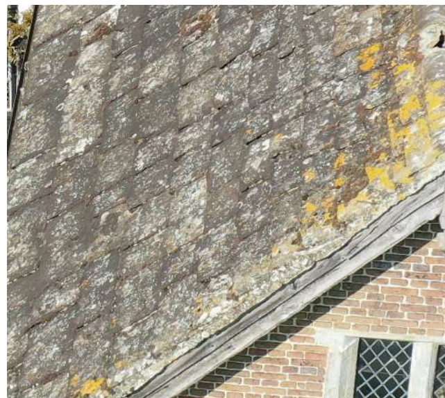
single lap diminishing HSS roof covering
