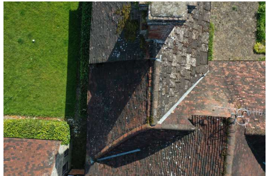
lead valley and abutments
