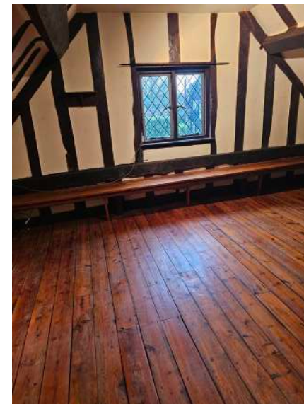
attic room to west gable
