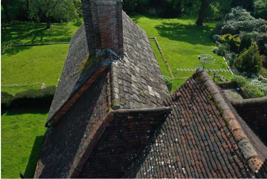
abutment of C15th roof to C17th roof
