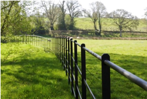
R1 - PERIMETER RAILING: ESTATE RAILING H:1000mm
