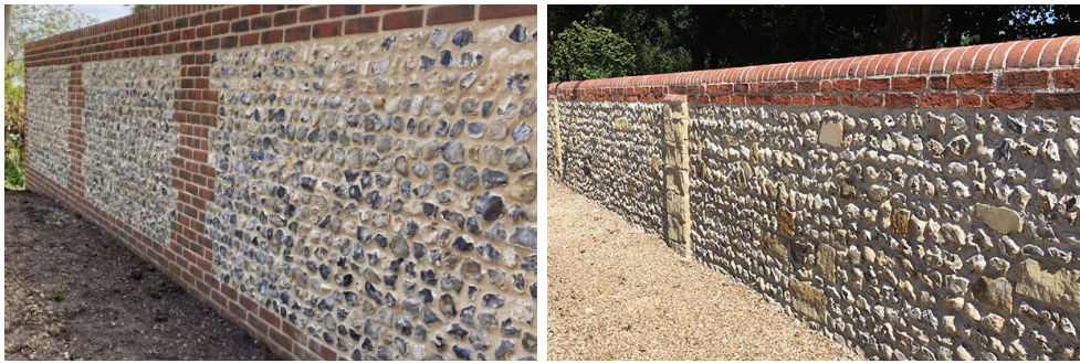
FLINT AND BRICK WALL 2.5 METRES HIGH
