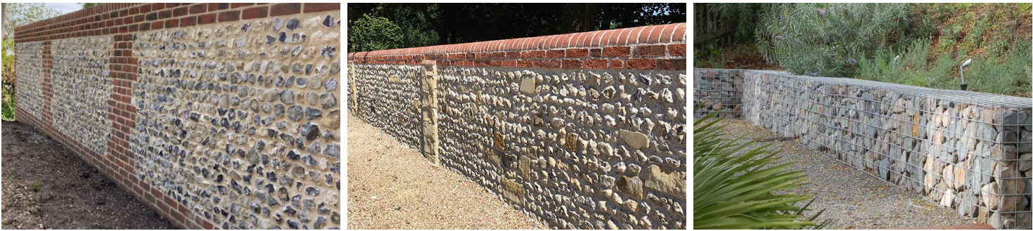
W1 - FLINT AND BRICK WALL HD: 2500x500mm
