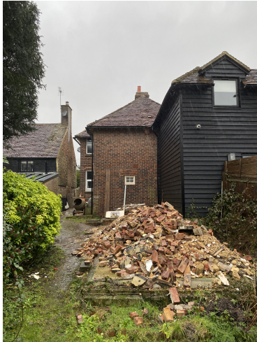
Photo of the rear facade and location of the proposed extensions
