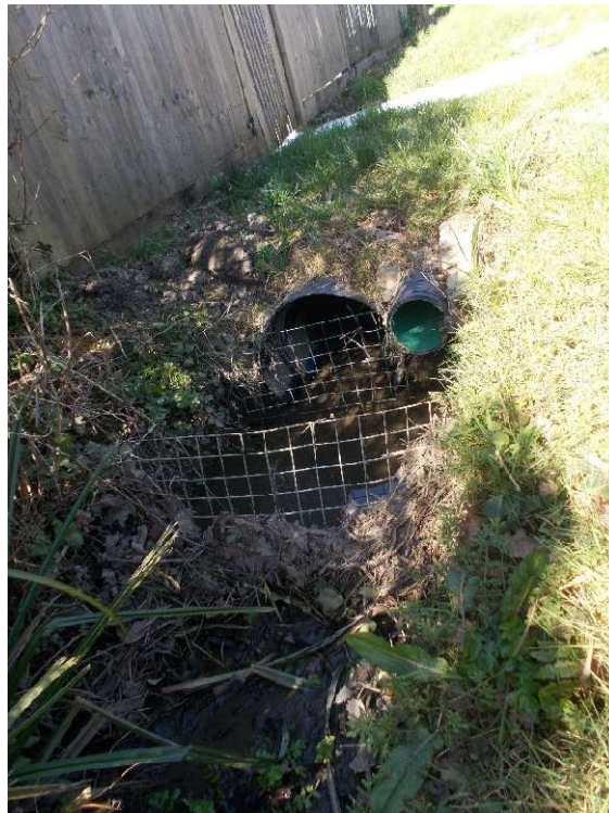
Culvert in Truslers Hill Lane
