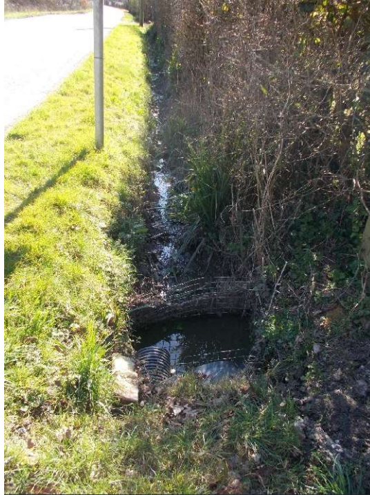
Drainage Ditch to the near/west side of Truslers Hill Lane
