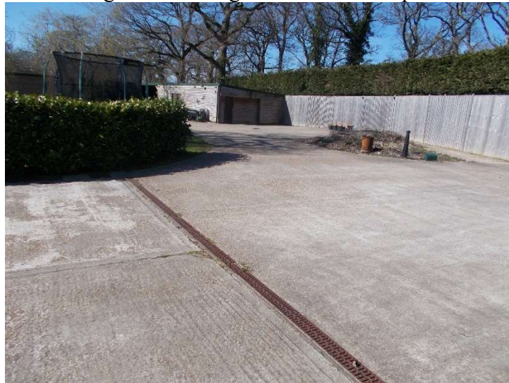
Parking area showing surface water strip drains
