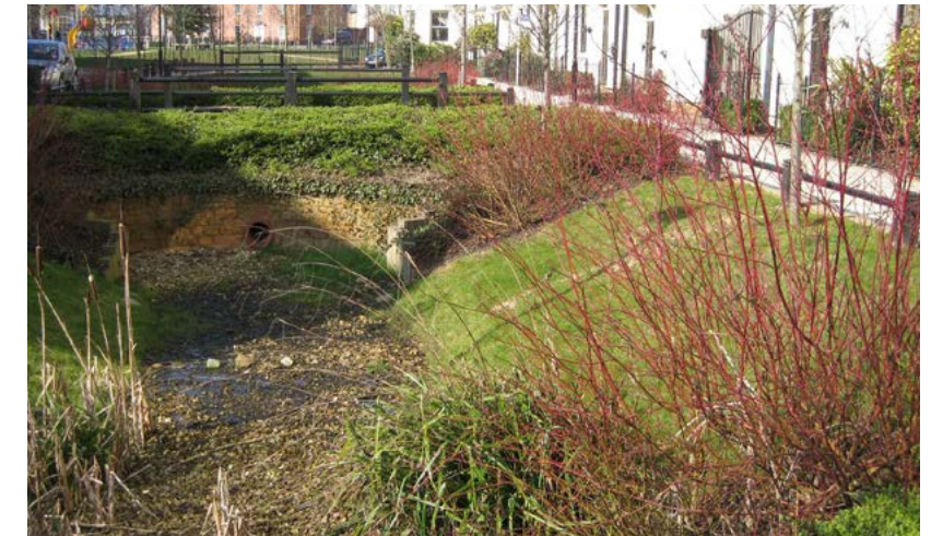
Surface water drainage can become a landscape feature of informal open space
