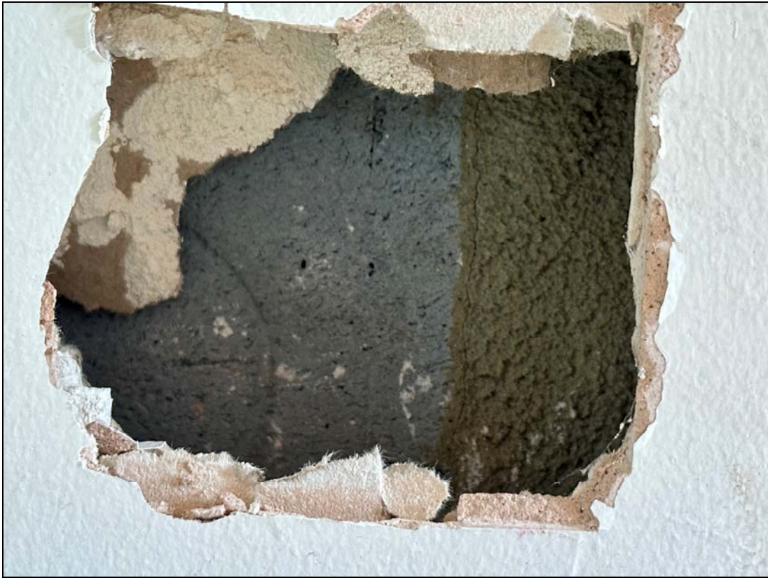
Plate 3: Detail of the block-work revealed behind the modern plaster board dry-lining system
