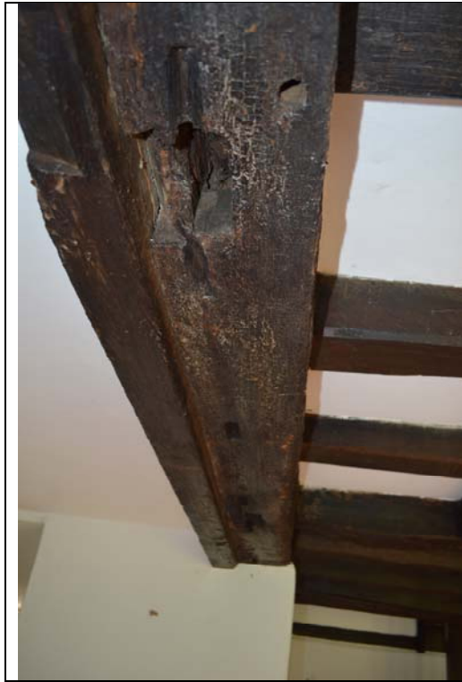
Plate 4: The two adjacent beams at the junction of bays 3 and 5
