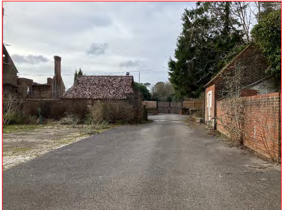
Plate 5 Edwardian walls and ancillary buildings to Horncastle House (now demolished) from entrance (dir. west)
