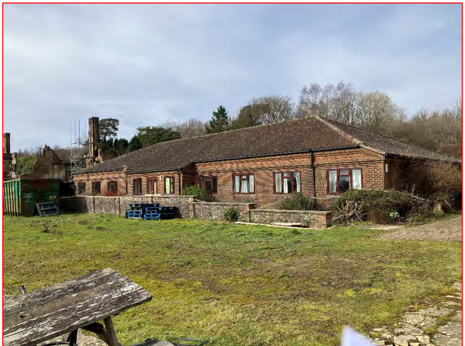
Plate 7 Modern structures of the former nursing home (dir. east)
