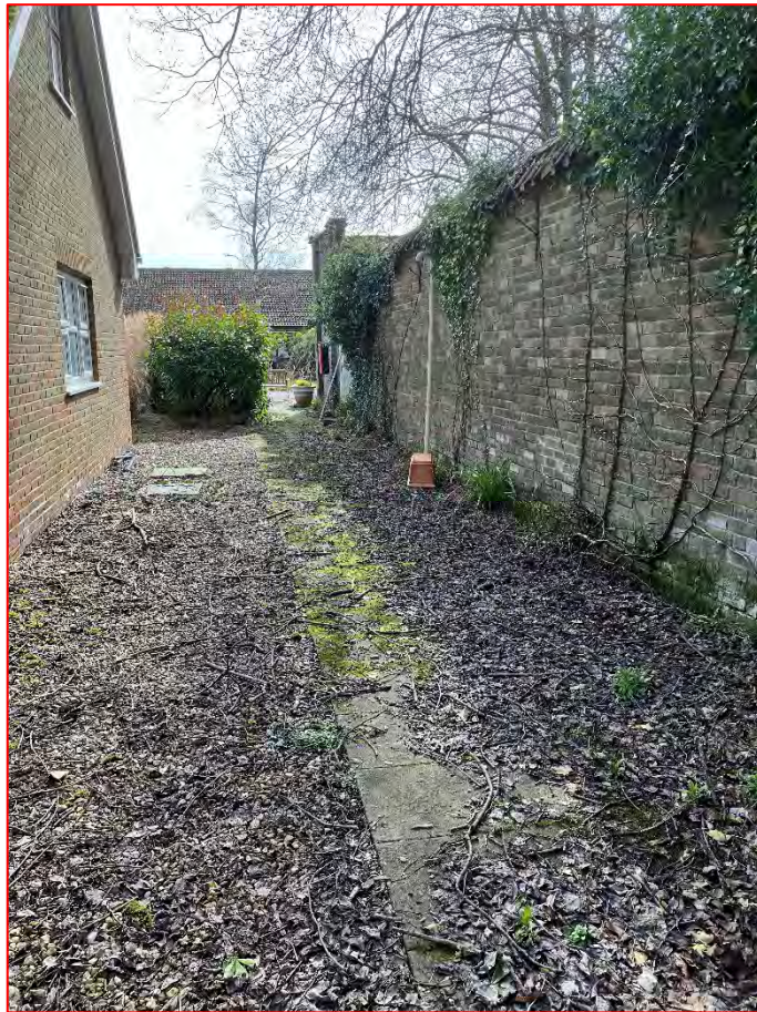
Plate 6 Garden walls along northern edge of property boundary to the now demolished Horncastle House
