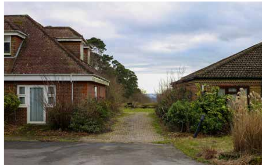
Image F: The view from the central courtyard to the south
