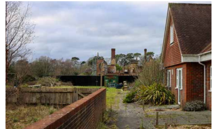
Image G: View of the derelict Horncastle House
