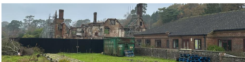
Figure 7: View of main house and extension from the rear (south)
