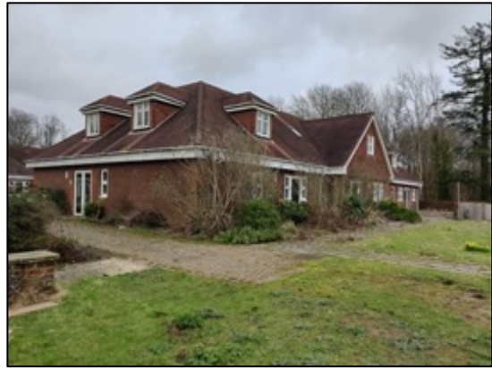
Photo 16: Southern elevation of building B6, facing north-east.
