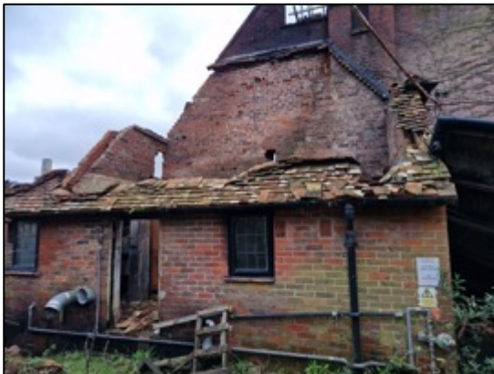
Photo 3: North-eastern elevation of building B1, facing south.
