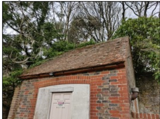
Photo 4: Southern elevation of building B4, facing north, showing woodland in the background.
