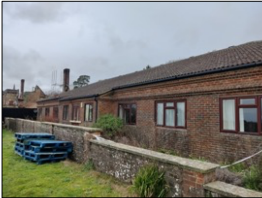
Photo 13: Southern elevation of building B2, facing north-west.
