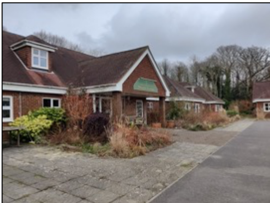
Photo 11: Southern elevation of the building B7, facing north-east, showing the hardstanding foreground.
