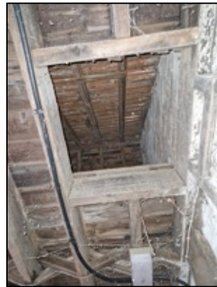
Photo 23: Internal aspect of building B3.
