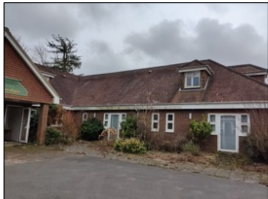
Photo 12: Northern elevation of building B6, facing south, showing the hardstanding in the foreground.
