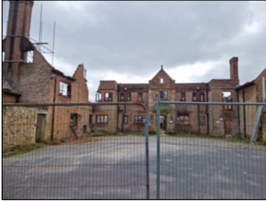
Photo 1: Northern elevation of building B1, facing south, showing hardstanding in the foreground.
