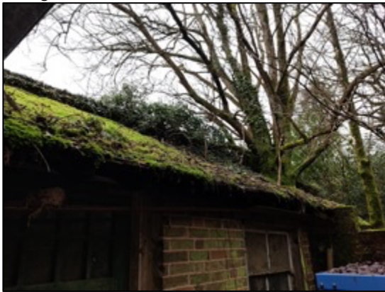
Photo 9: Northern elevation of building B5, facing south-west.
