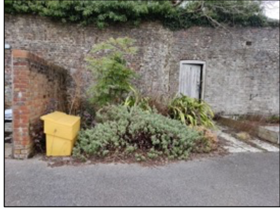
Photo 8: Southern elevation of building B5, facing south, showing the hardstanding in the foreground.
