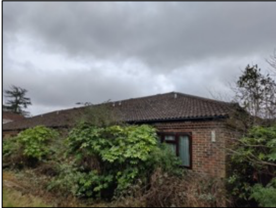
Photo 7: Northern elevation of building B2, facing south, showing the introduced shrub in the foreground.
