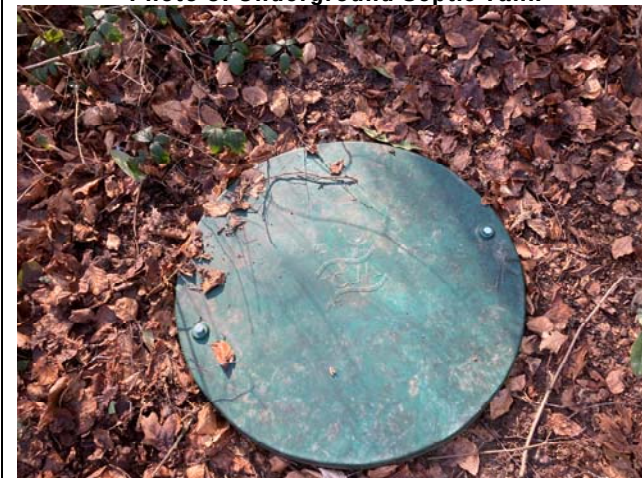
Photo 3: Underground Septic Tank
