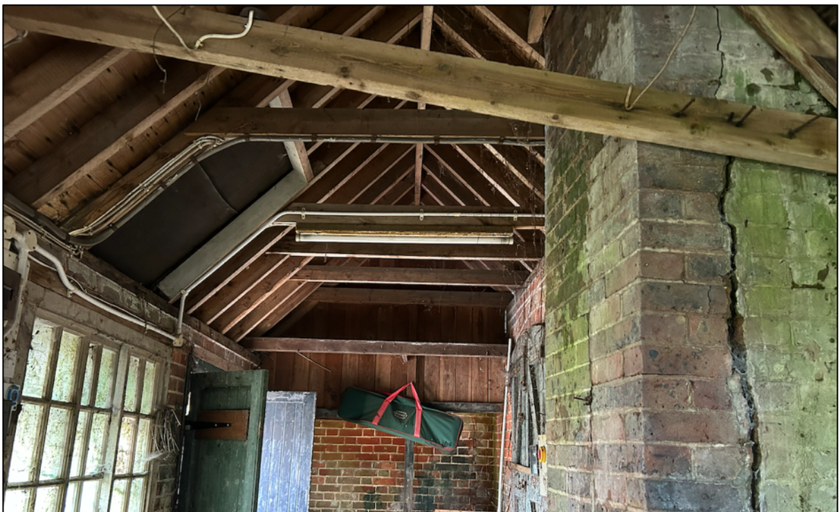
Photograph 6. The internal aspect of the shed, which is open to roof height and well lit.
