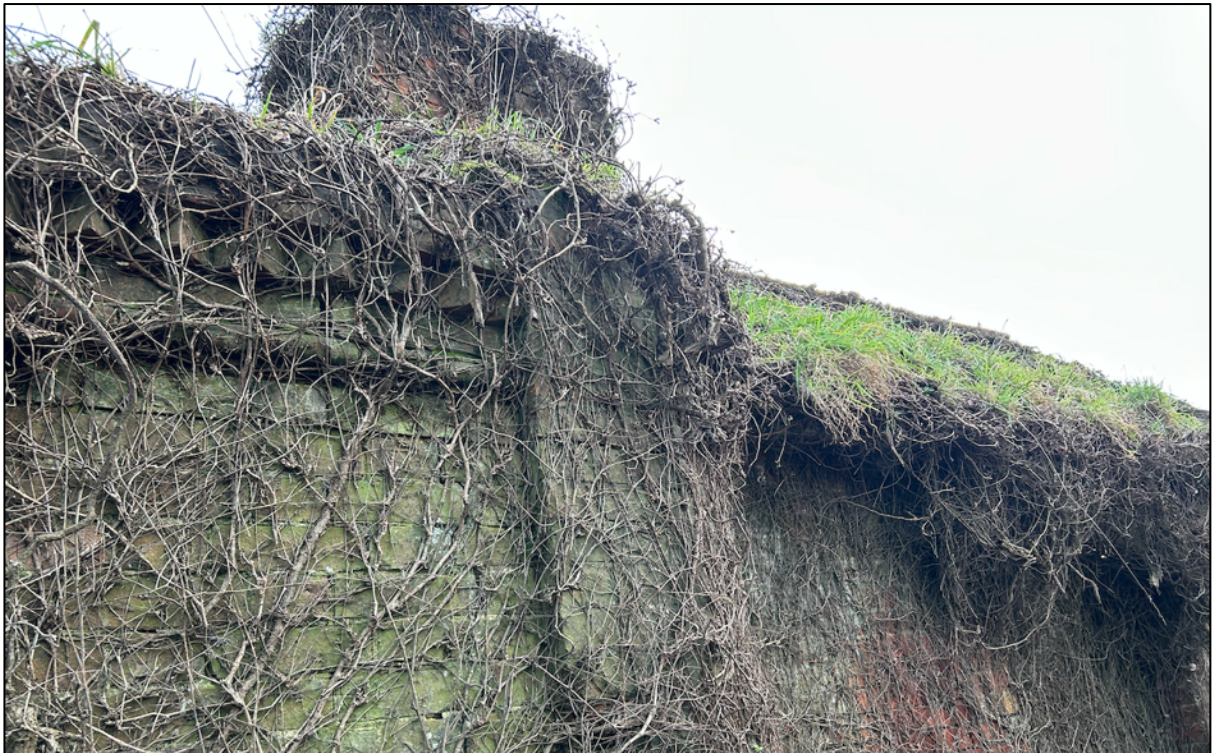
Photograph 2. A restricted view of the western face of the shed, which sits directly adjacent to the B2028
