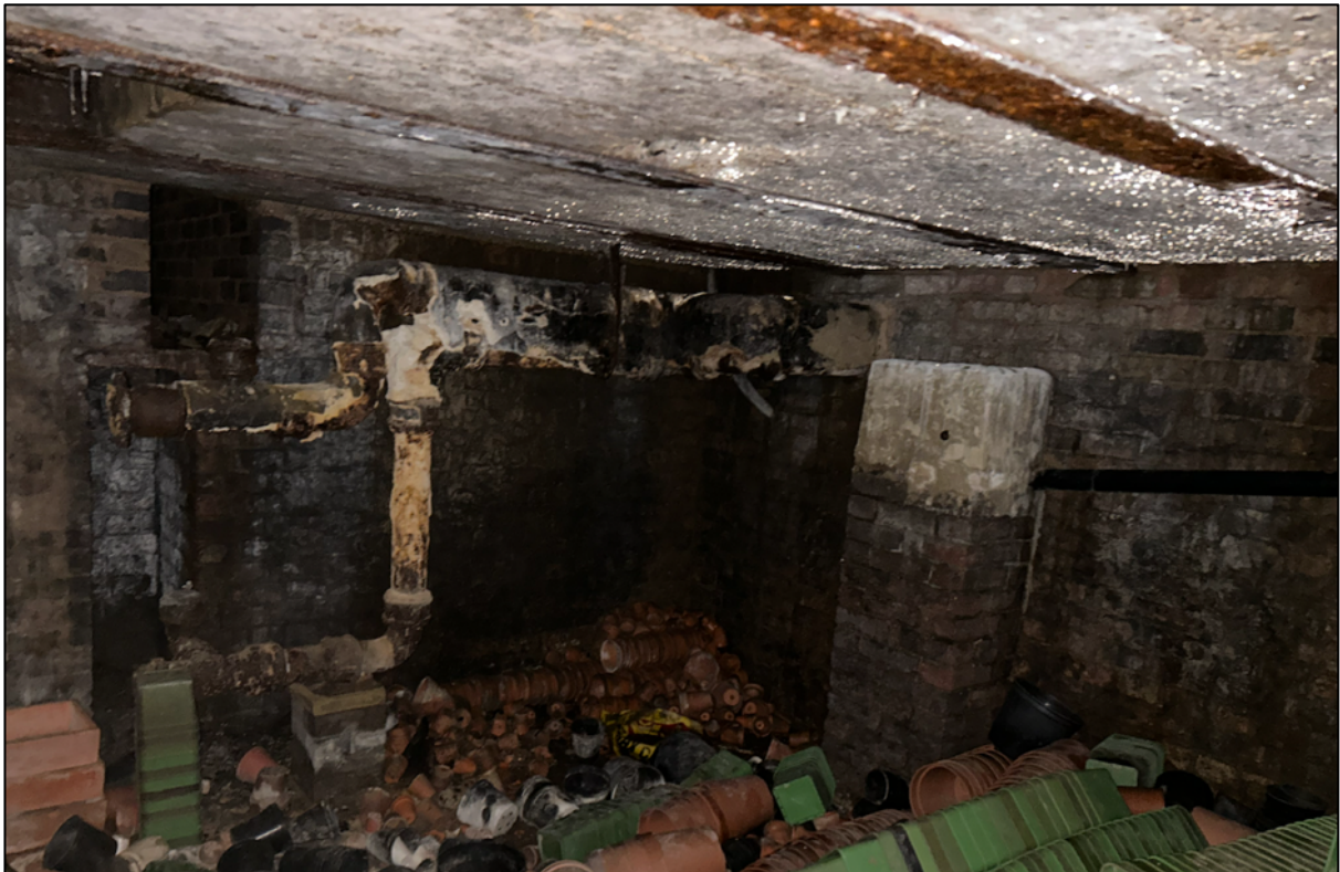
Photograph 4. An underground area understood to have formerly been used for heating a greenhouse.
