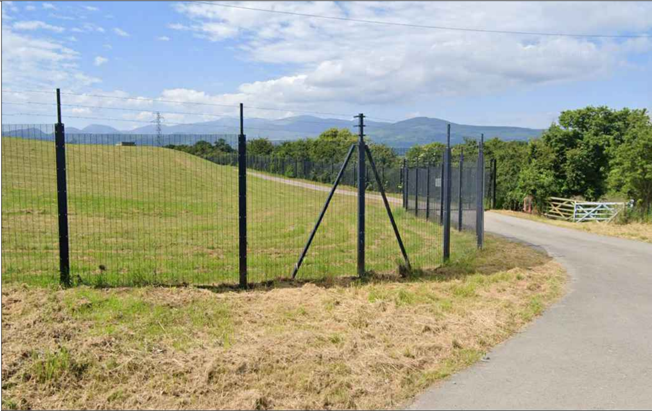
Covered reservoir from Streetview capture © 2025 Google Image illustrates typical installation of a steel welded mesh fence (unknown product and rating). Note the raking braces for the corner straining post and the thin extension pieces carrying three strands of barbed wire over. Panels stepped to accommodate ground profile
