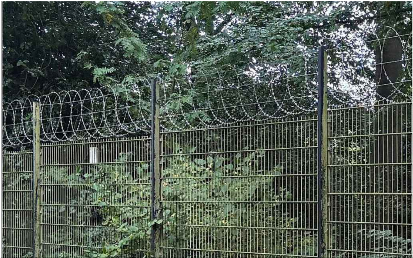
Image from MFD Communication Infrastructure Ltd Image illustrates fence topping of flattened barbed wire concertina carried on three strands of barbed wire. Although this fencing product probably does not carry an LPS 1175 security rating of B3 (SR2), it does show the an installation of the preferred topping at a governmental secure site
