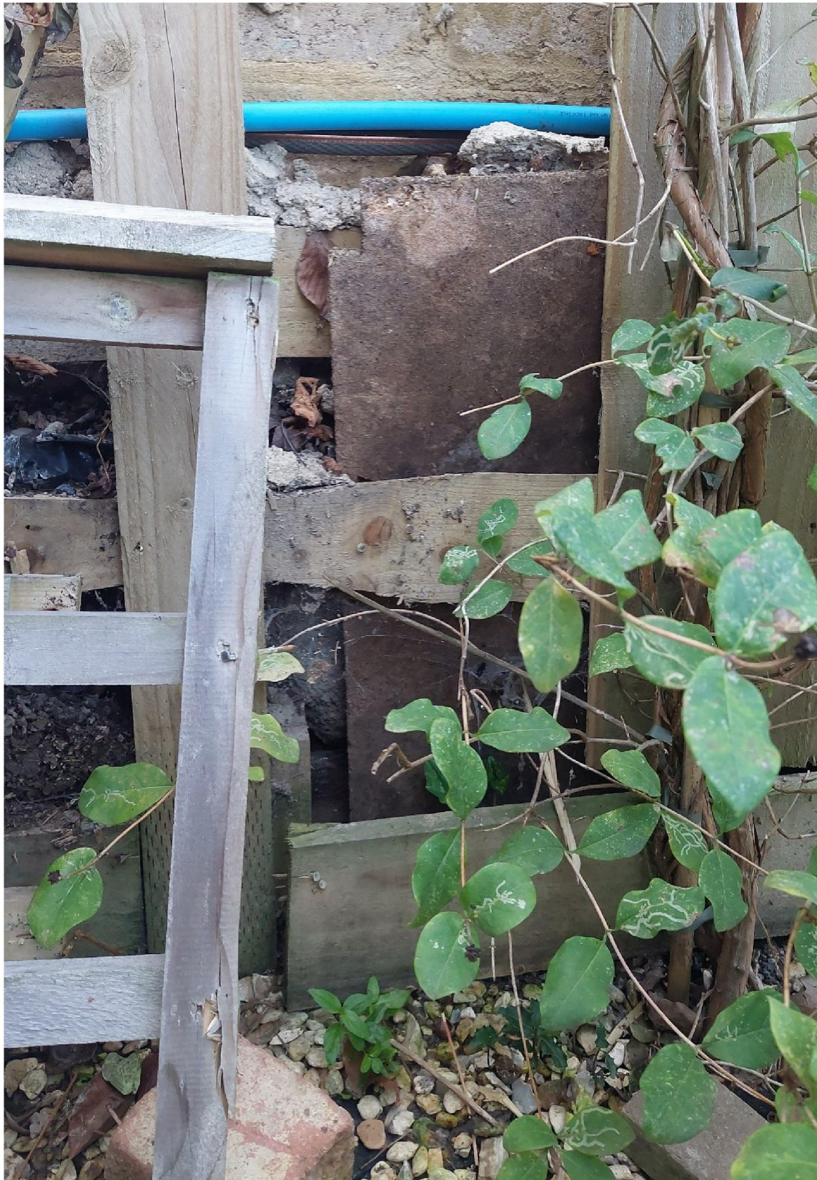
Figure 2: Piece of hardboard wedged between the original horizontal slats attached to the fence panel, and the newly installed horizontal board above (behind the hardboard).
