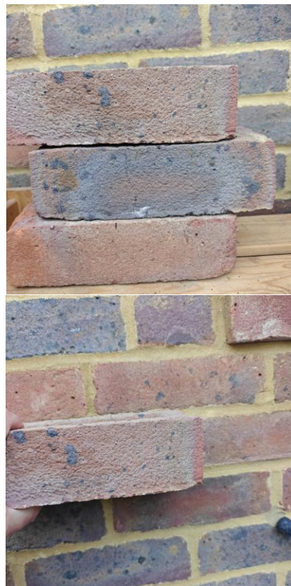
Actual Michelmersh samples compared directly with existing wall
