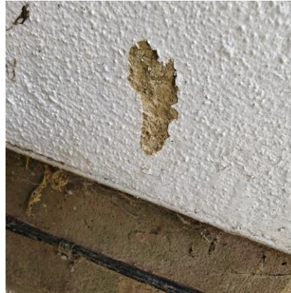
Existing white paint over sandy cementitious render; exposed area photographed
