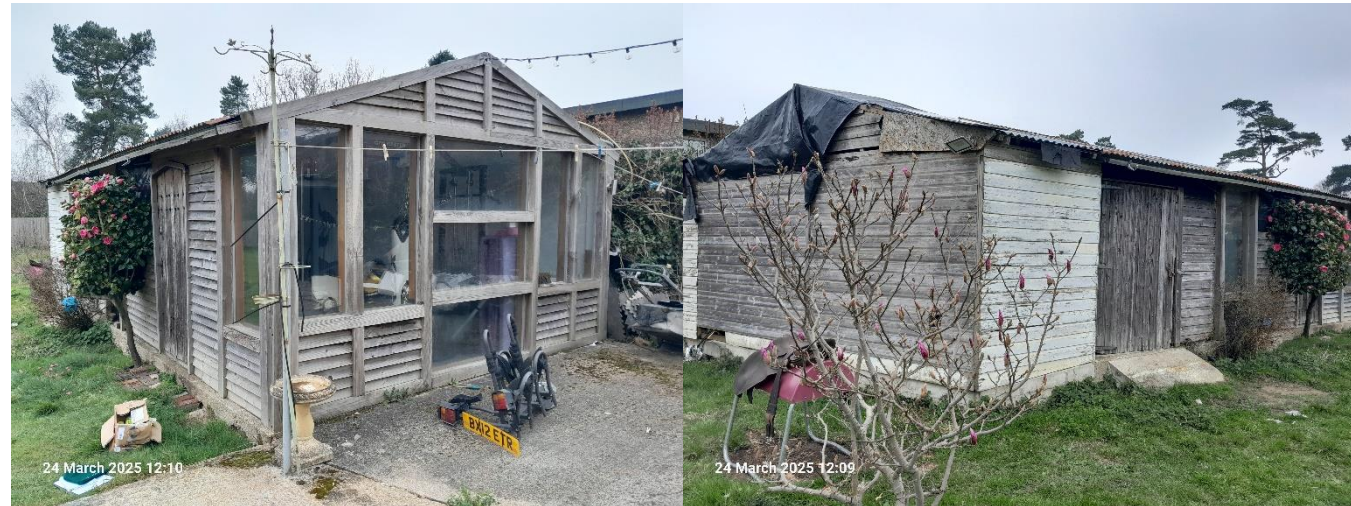
B2: Southeastern elevation (left) and southwestern elevation (right).
