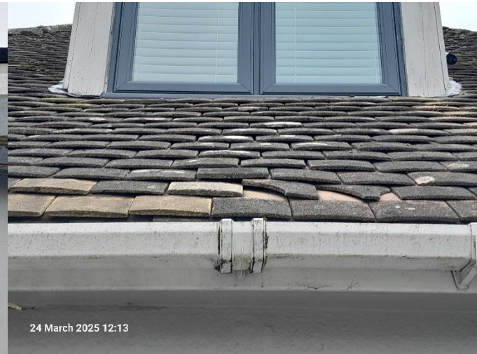
B1: Well sealed eaves and tight fitting windows (left) and lifted and broken roof tiles (right).
