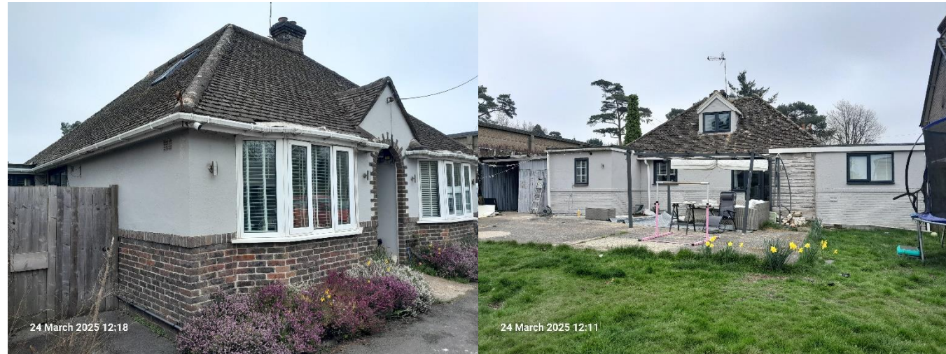
B1: Southeastern elevation (left) and western elevation (right).
