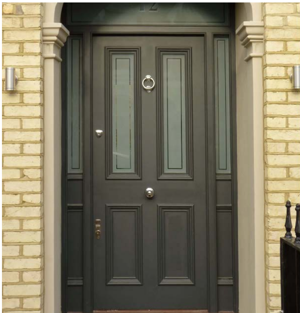
Front Doors with glass panelling.
